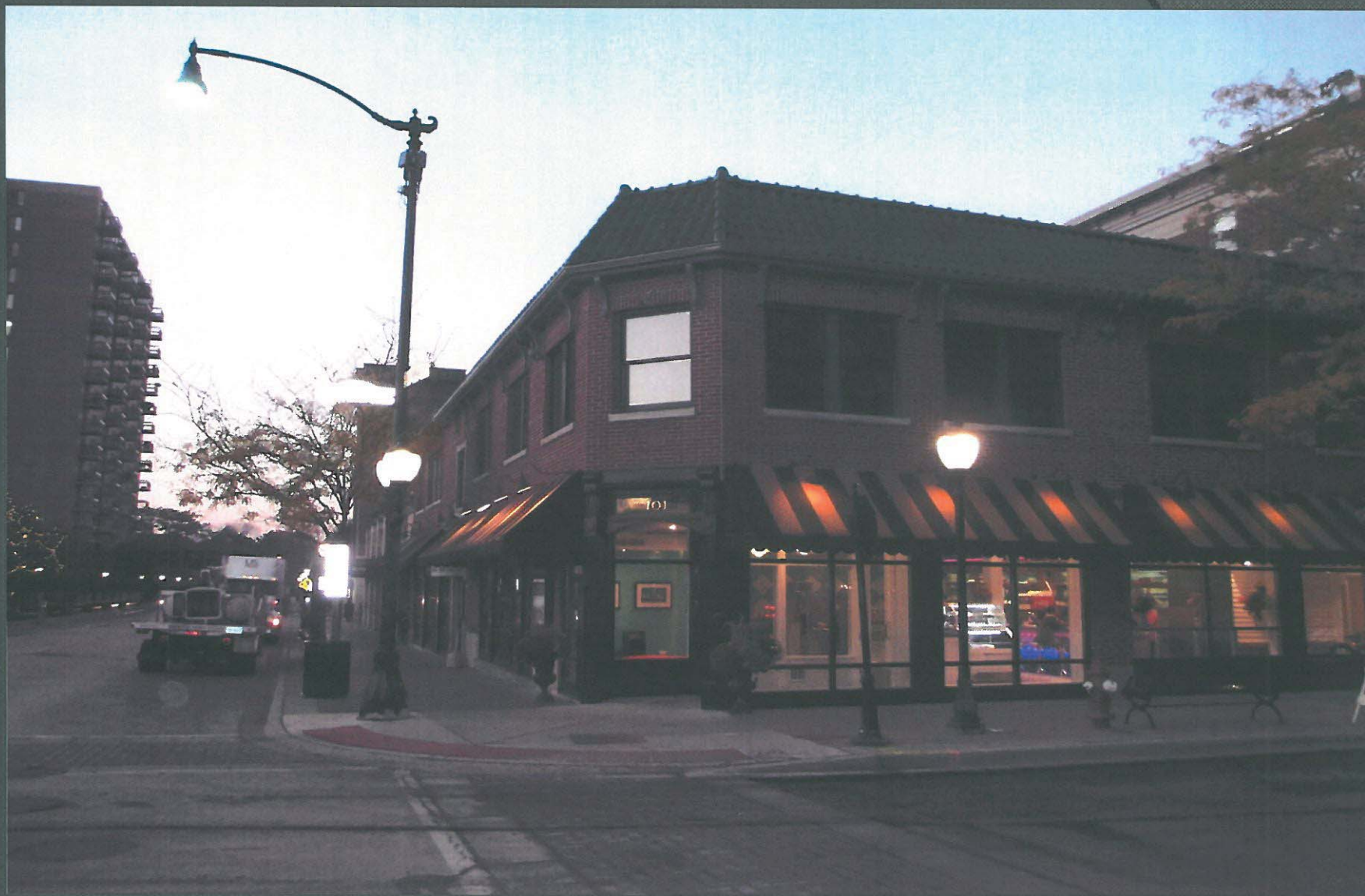
101 West Campbell Street
