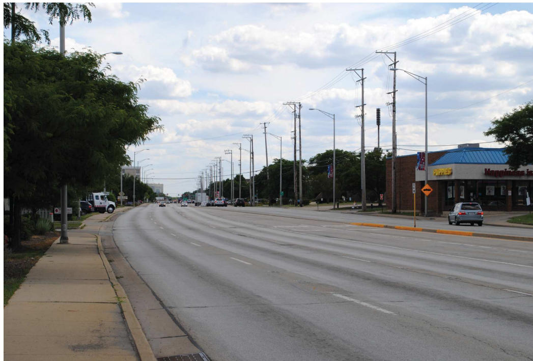
Existing Conditions - Southbound Arlington Heights Road at Golf Road
