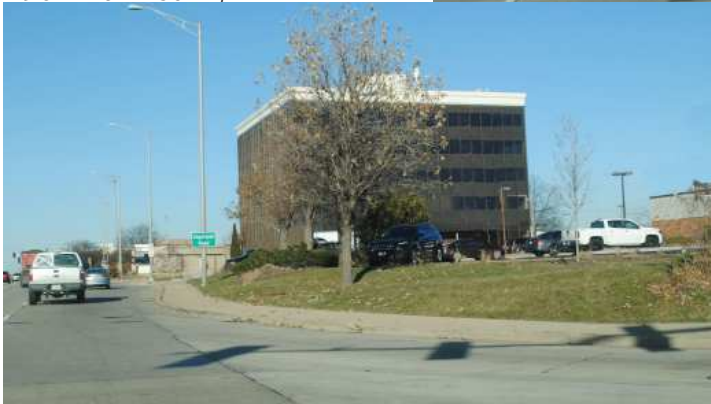
I-90 Exit Existing
