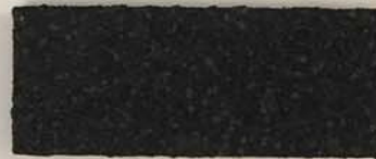
ASPHALT ROOF SHINGLES
