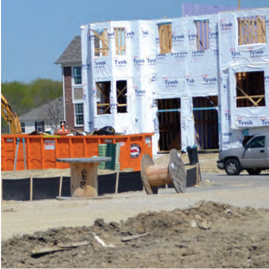
Sheffield Square Construction, Orland Park
