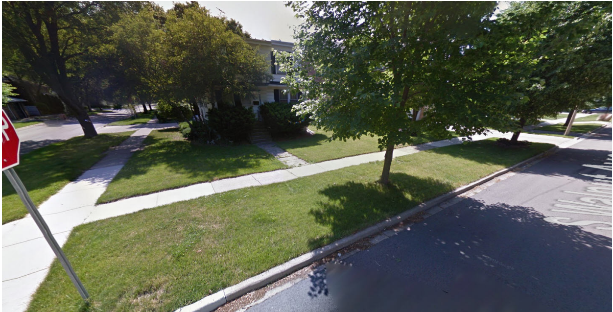
Photograph of Existing Structure
