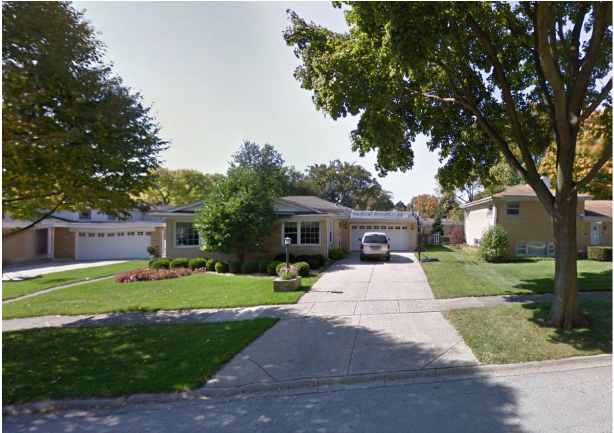
Photograph of Existing Structure
