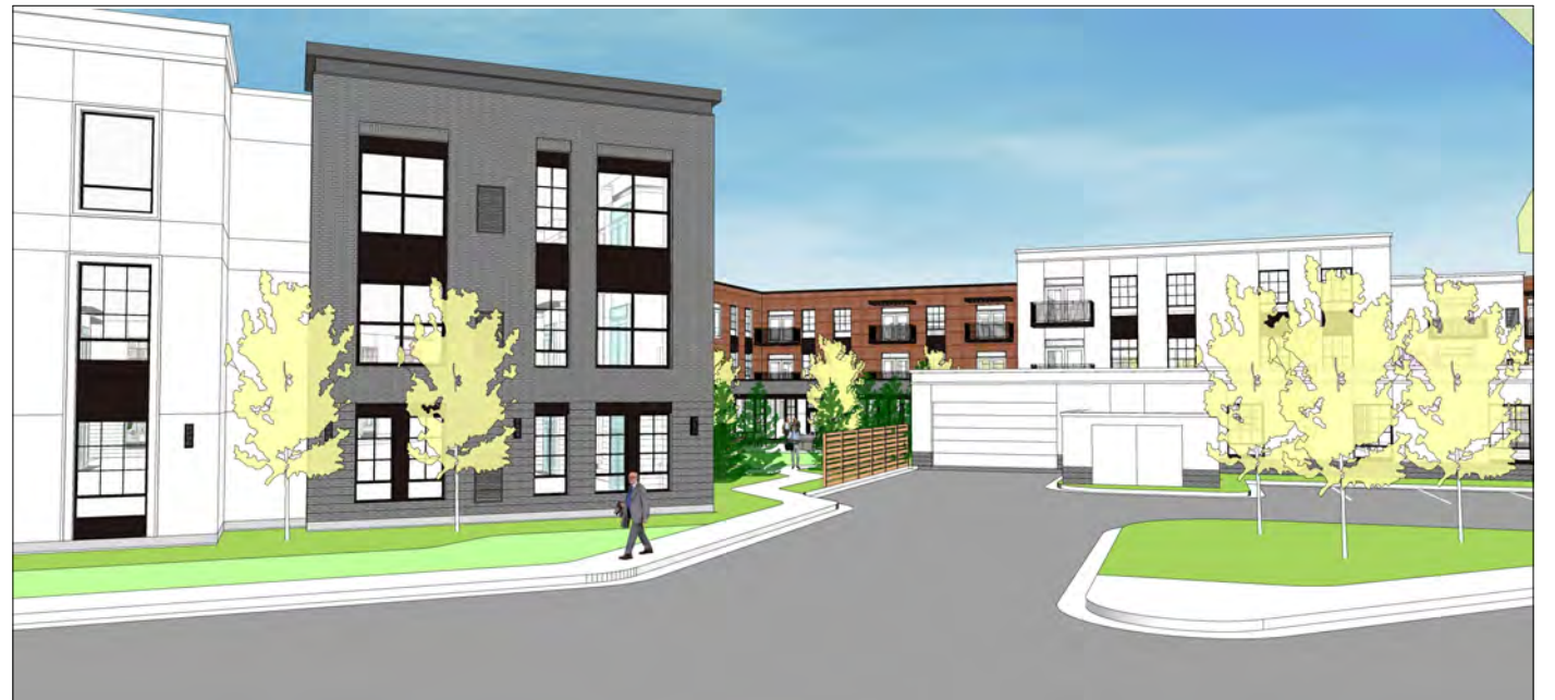
PEDESTRIAN VIEW ALONG TONNE DR
