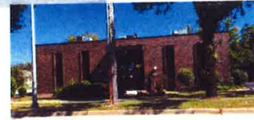
2 nd bldg. south
