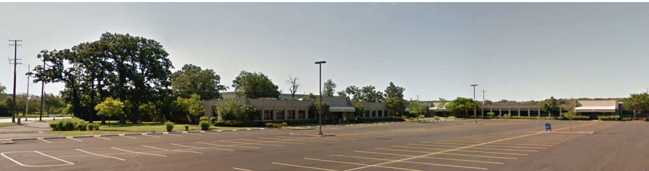
EXISTING BUILDING - NORTH
