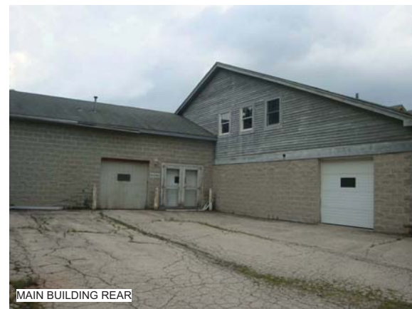
VACANT RESIDENCE ON PROPERTY - LOOKING NORTH
