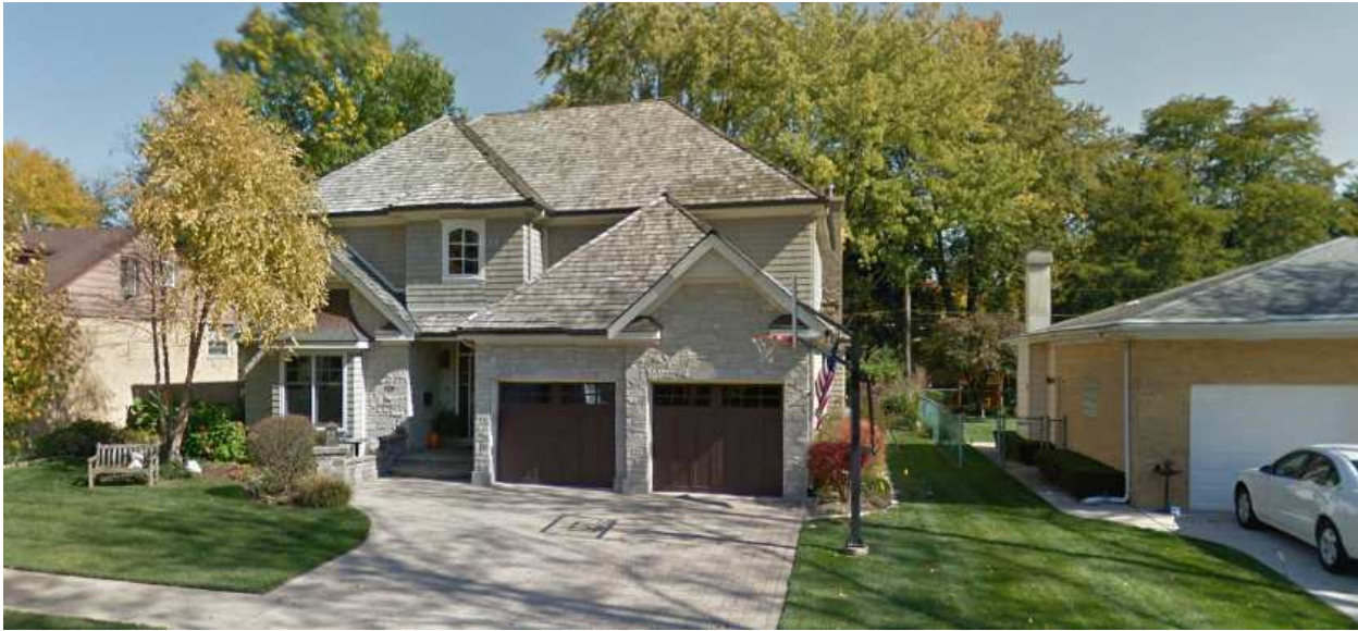
Image 1, 519 S. Donald Avenue. The hipped roof forms, single story elements, and neutral color palette help this larger scale home to blend into the neighborhood.
