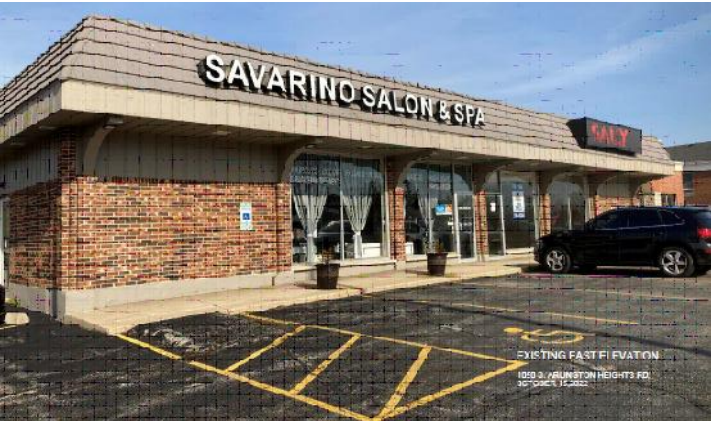
EXISTING EAST WALL PHOTO
