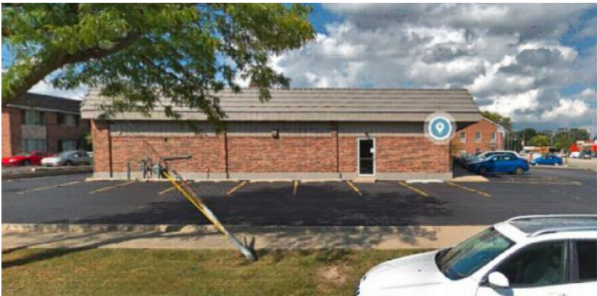
EXISTING SOUTH WALL PHOTO
