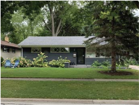
509 S. PHELPS AVENUE DIRECTLY ACROSS ST.
