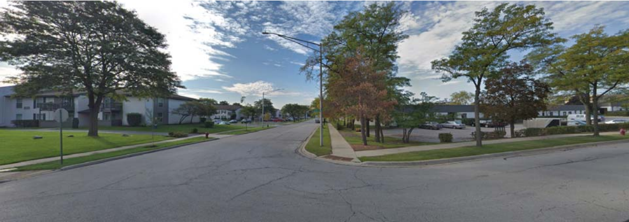
5 STREET VIEW - FROM NE CORNER, LOOKING SOUTH
