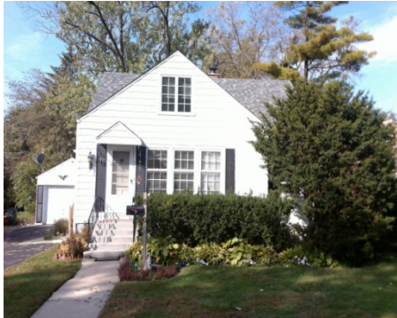
PROPERTY ACROSS 2 810 N PINE AVE
