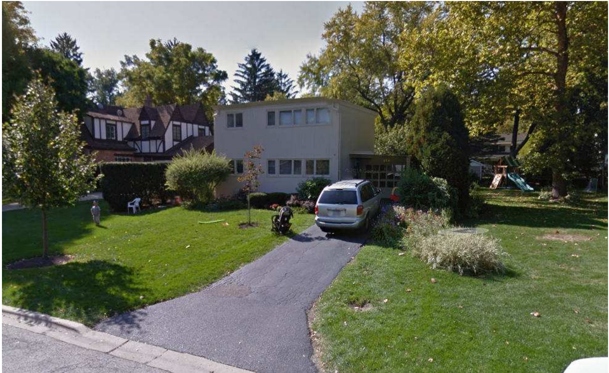
Photograph of Existing Structure
