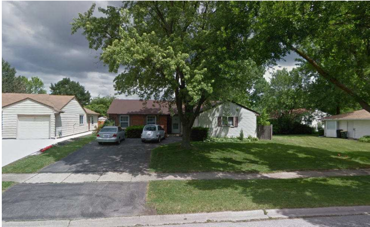
Photograph of Existing Structure
