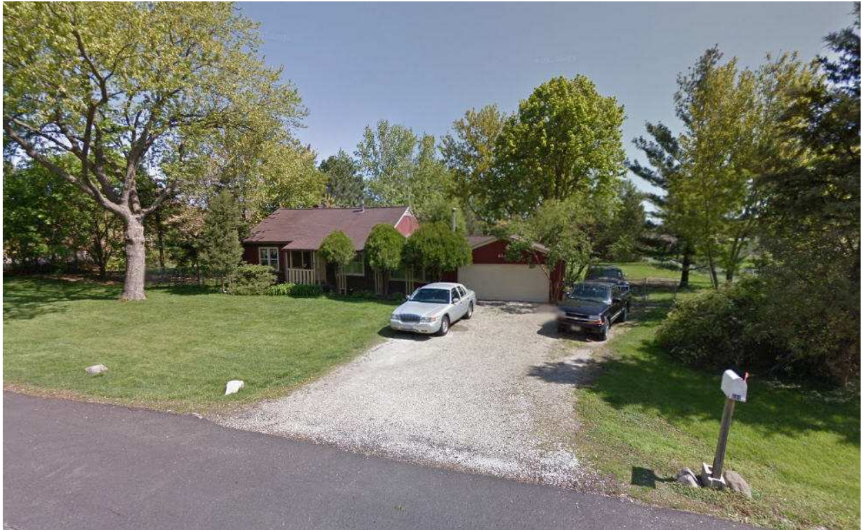
Photograph of Existing Structure
