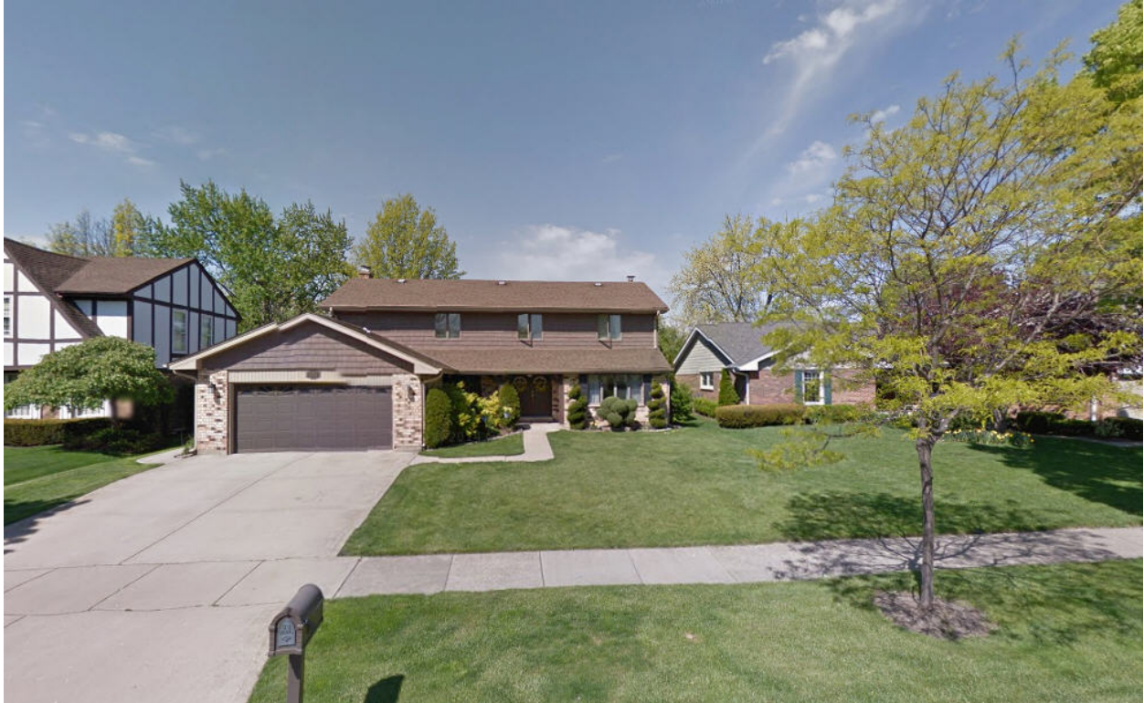
Photograph of Existing Structure
