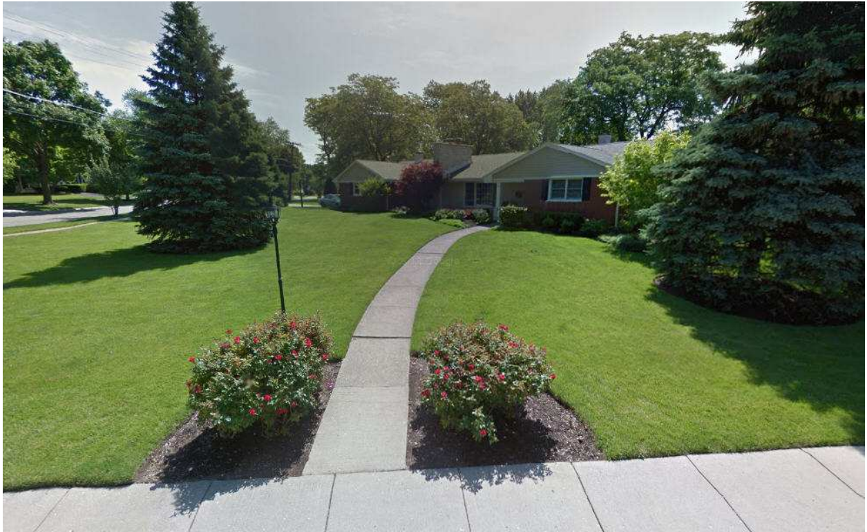
Photograph of Existing Structure
