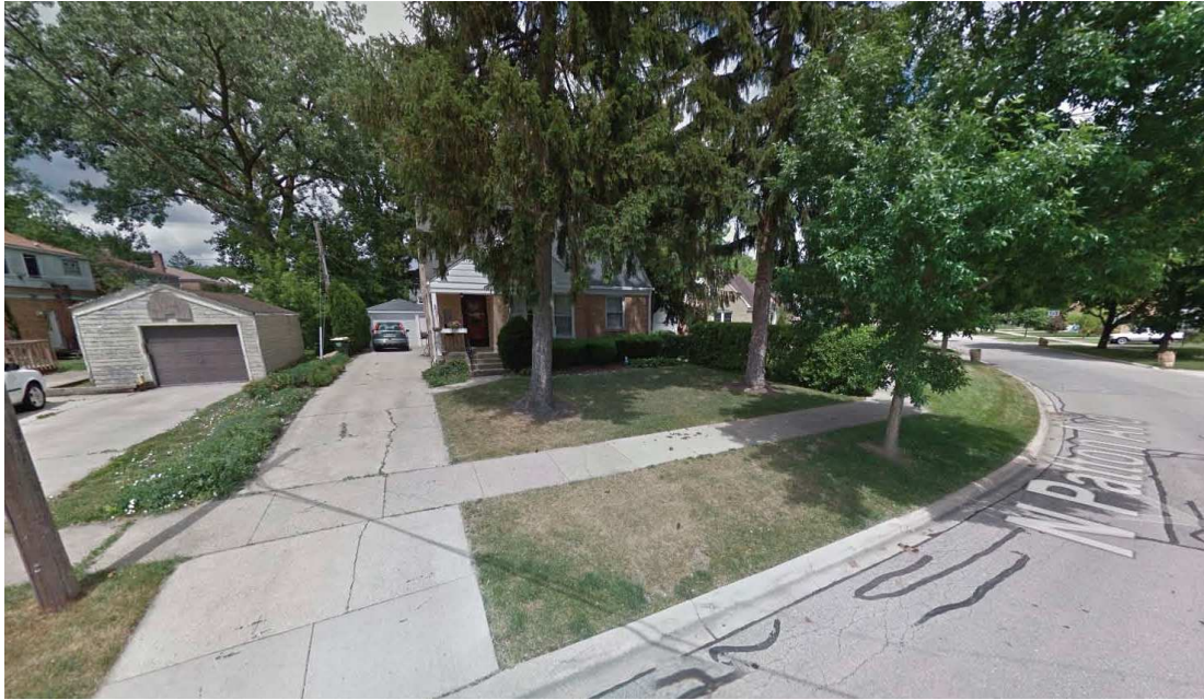
Photograph of Existing Structure
