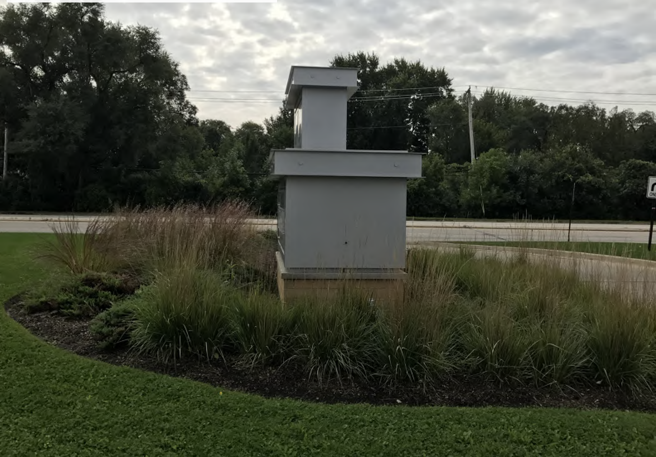
Existing Euclid Sign Looking South
