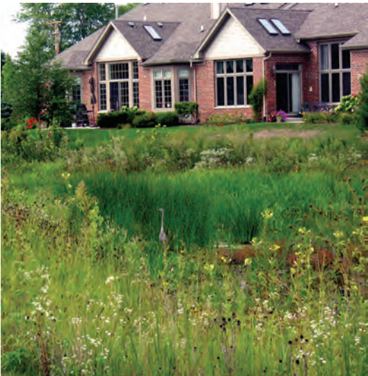
Evergreen View Detention Facility, Orland Park
