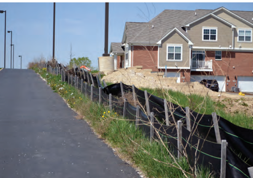
Sheffield Square Silt Fence, Orland Park
