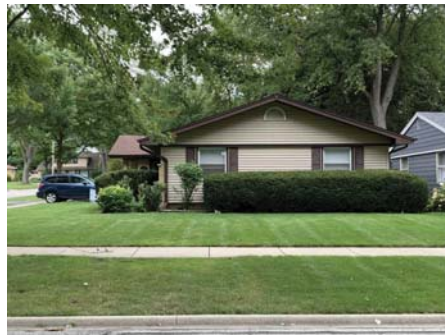
2105 E. PARK STREET 1 HOUSE LEFT ACROSS ST.
