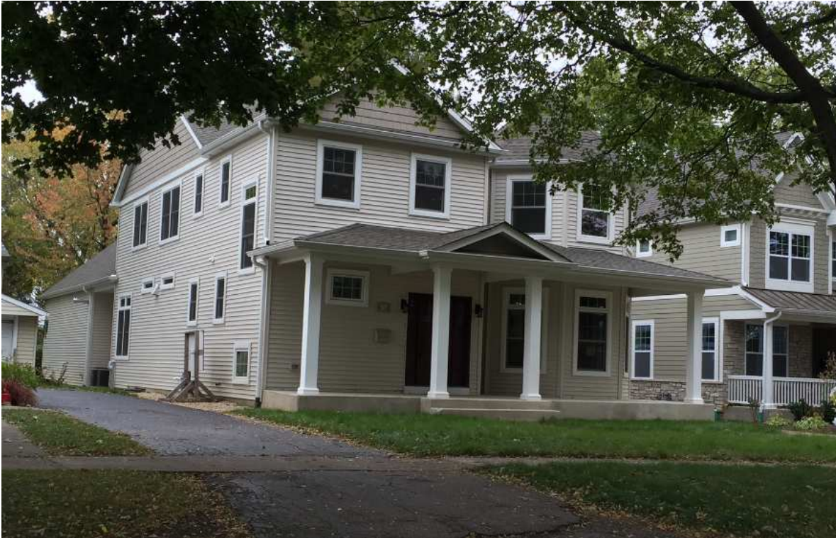
Image 2. 917 N. Beverly Lane, teardown 2011. Attached side load garage in rear of house.
