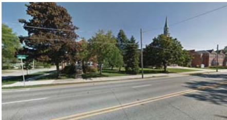
CHURCH PROPERTY ALONG ARLINGTON HEIGHTS ROAD
