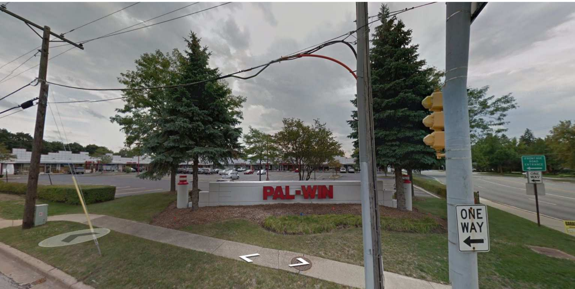
Existing Sign and Wall to be Removed
