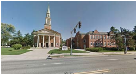
CHURCH PROPERTY ALONG ARLINGTON HEIGHTS ROAD
