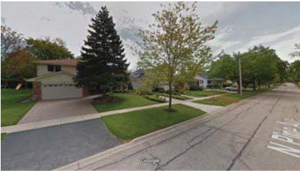
PROPERTY ACROSS FROM CHURCH ON PINE STREET
