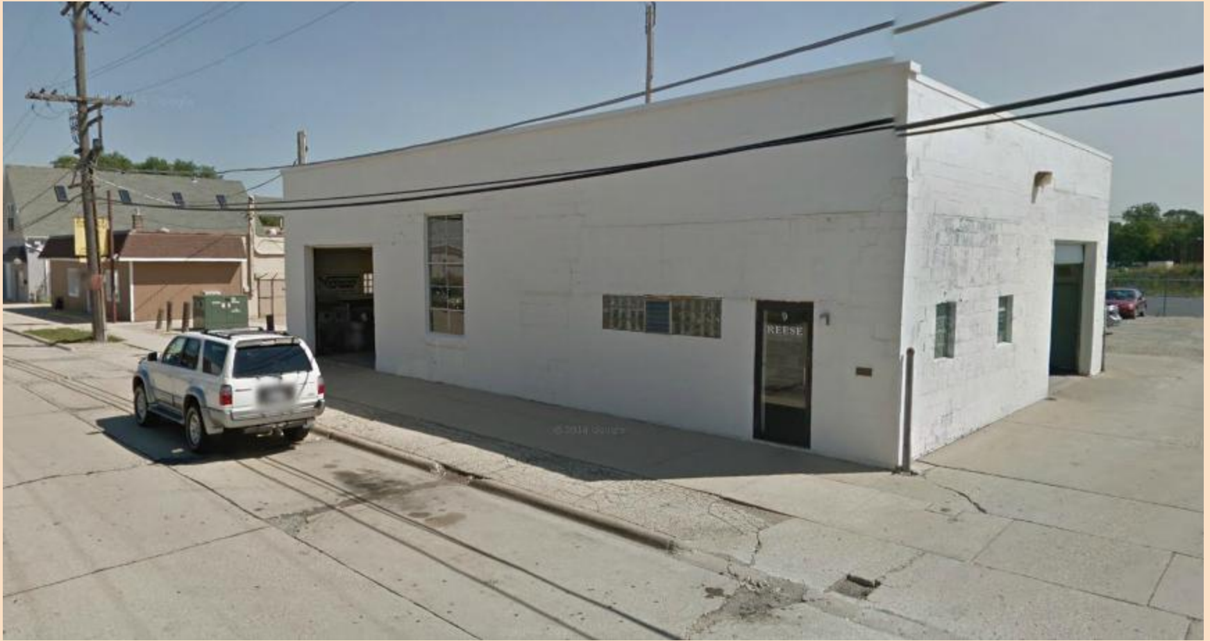
Looking East from Hickory Avenue
