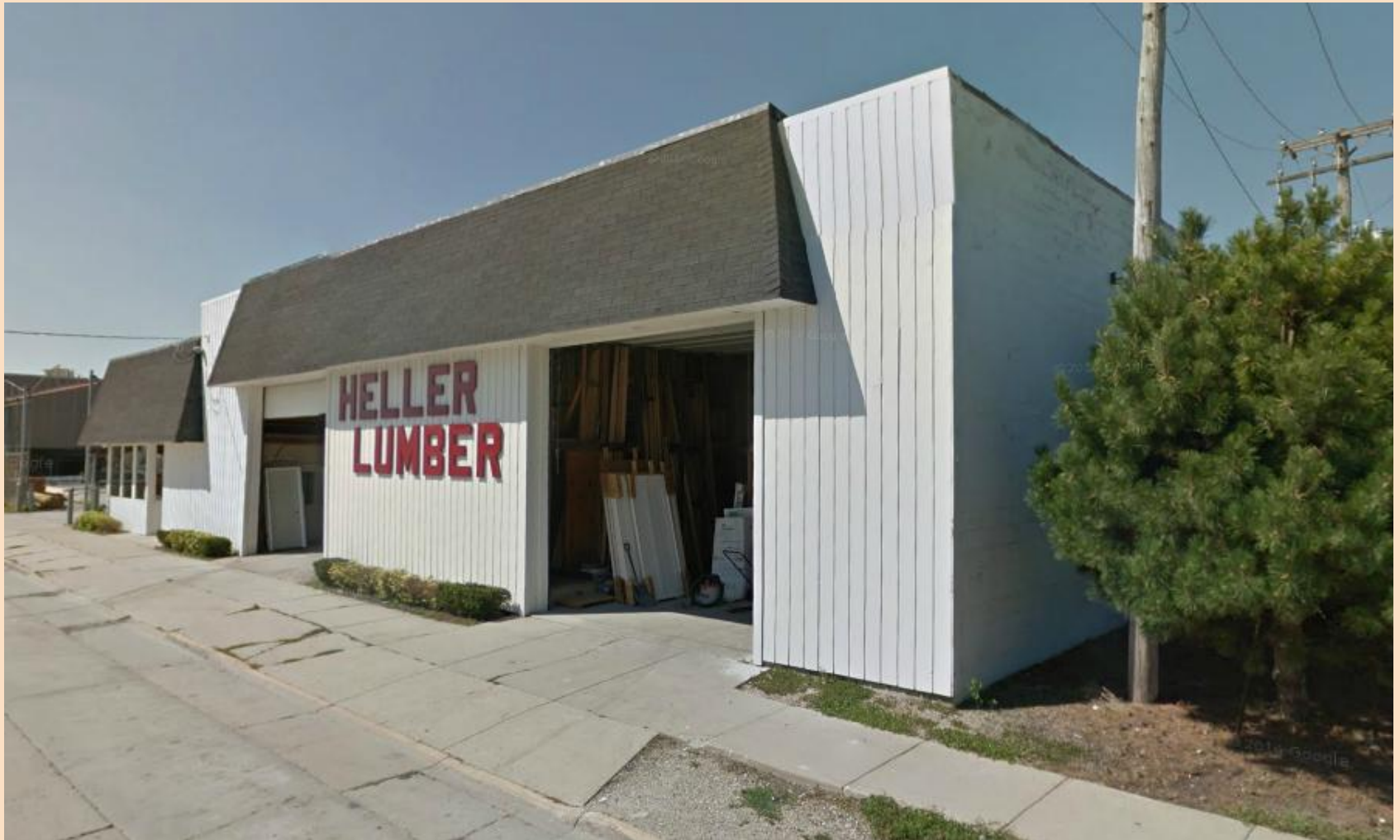
Looking Southwest from Hickory Avenue
