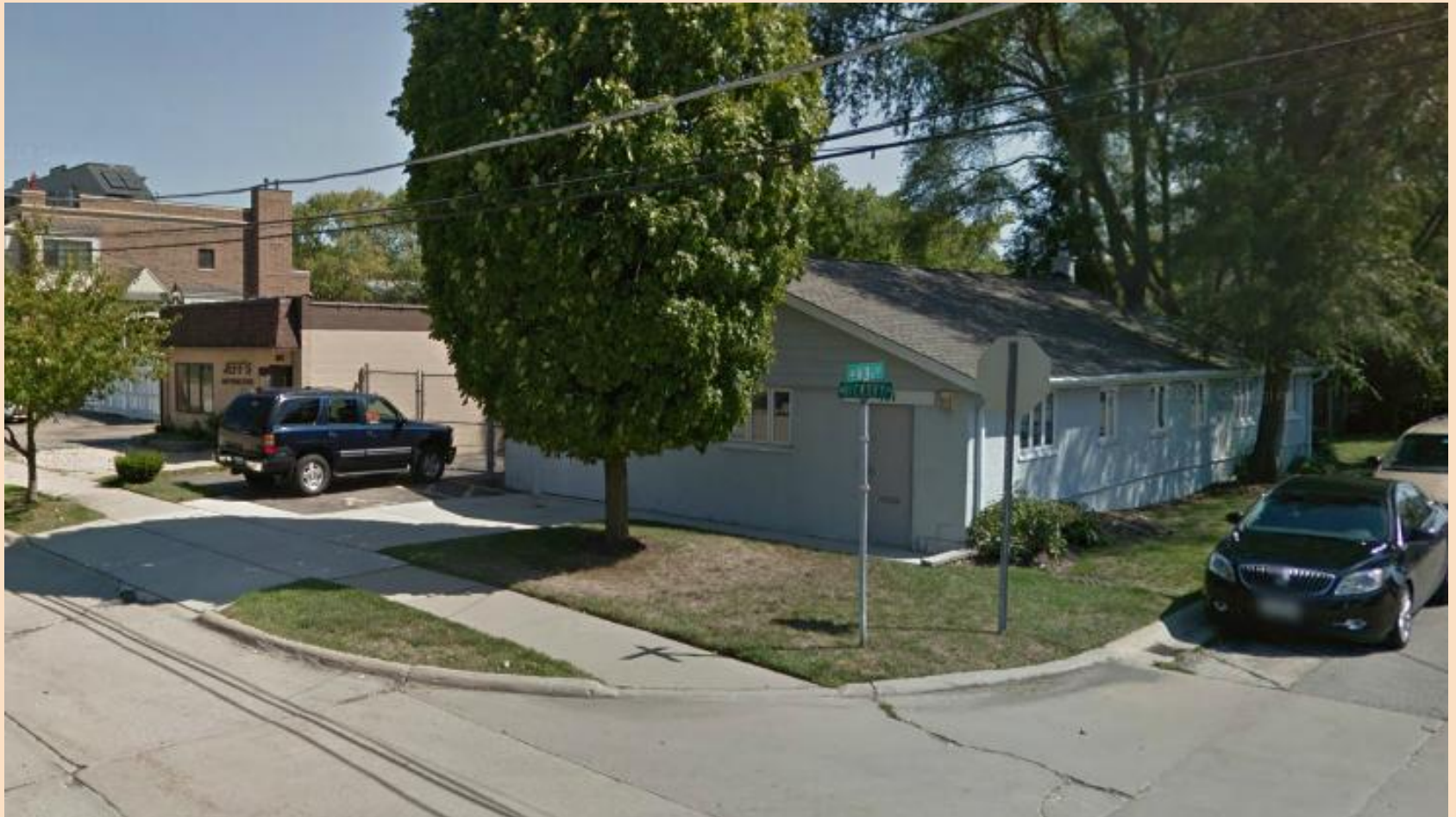
Looking East from Hickory Avenue
