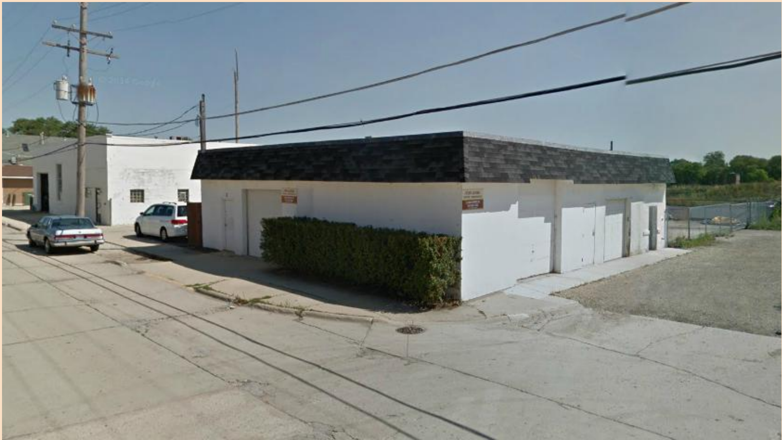
Looking East from Hickory Avenue
