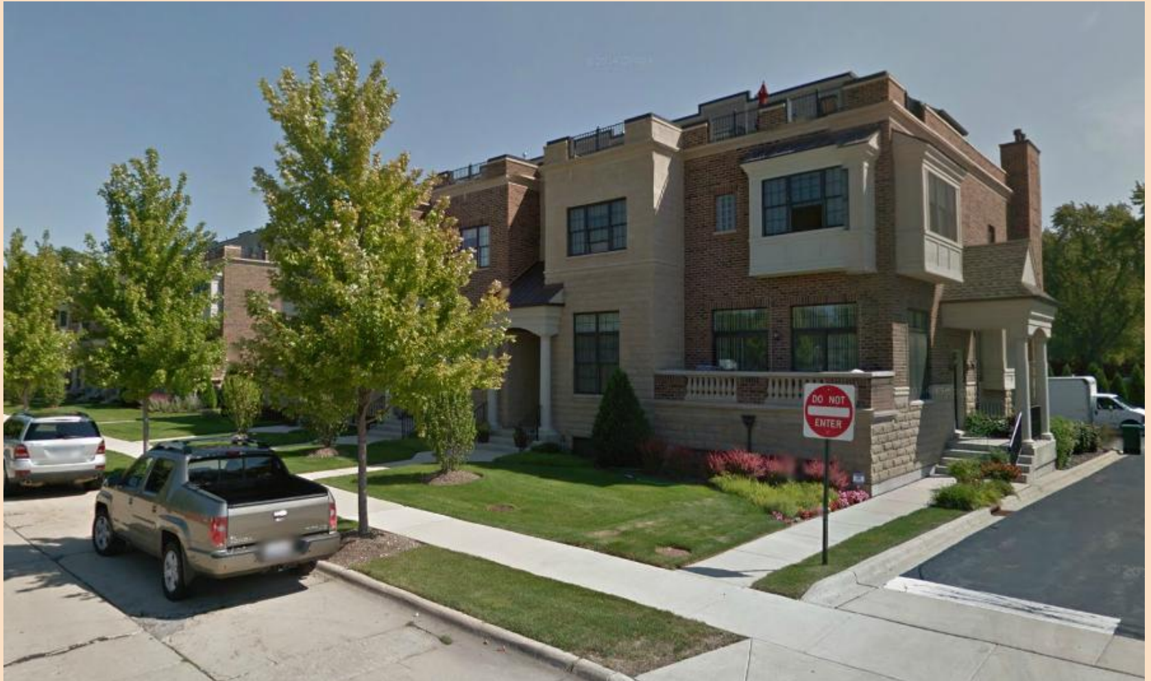
Looking East from Hickory Avenue
