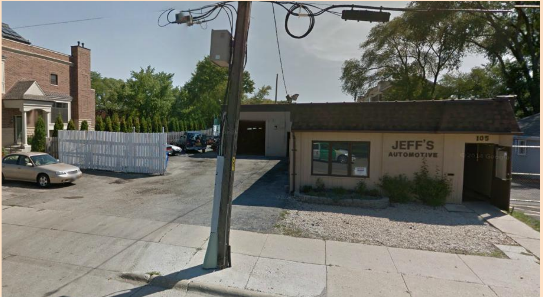
Looking East from Hickory Avenue
