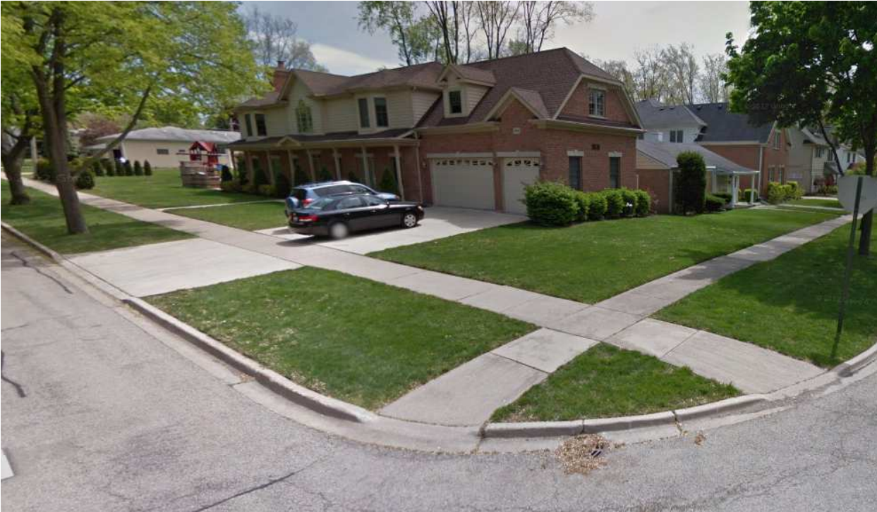
Image 1. 845 N. Hickory Avenue, teardown 2004. Attached garage facing the corner.
