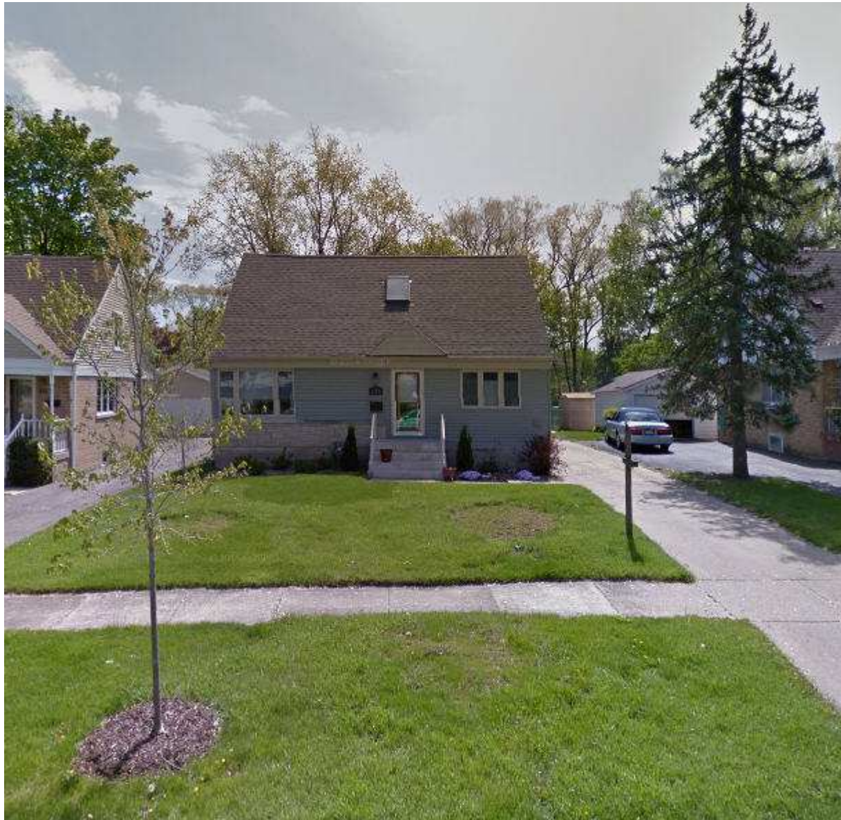
Photograph of Existing Structure
