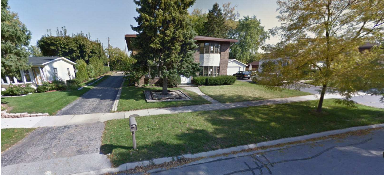
Photograph of Existing Structure
