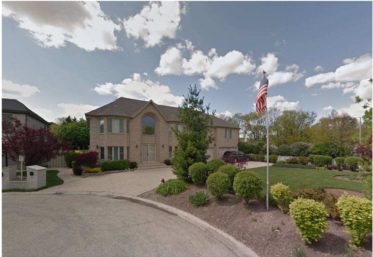
Photograph of Existing Structure
