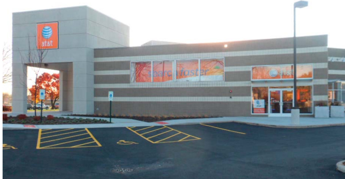
1 Main Entry - View from West parking lot near E. Palantine Rd.
