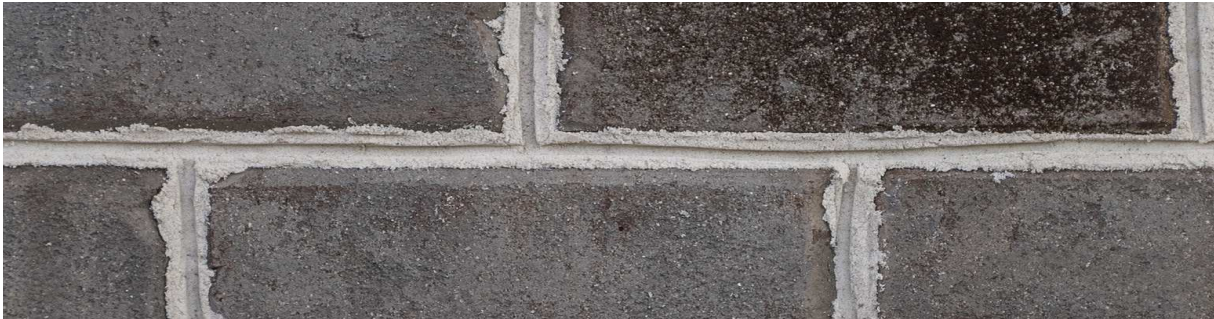
Brick Chimney – Palmetto Ashland
