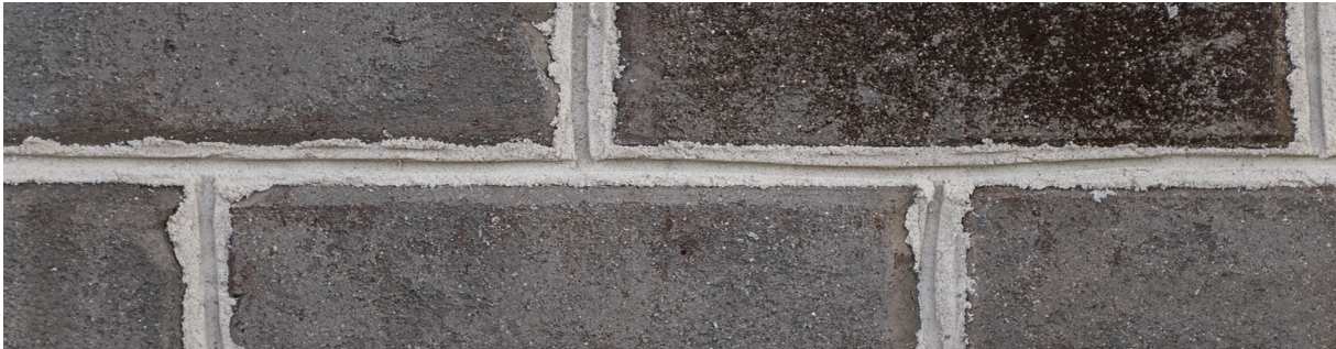
Brick Chimney – Palmetto Ashland
