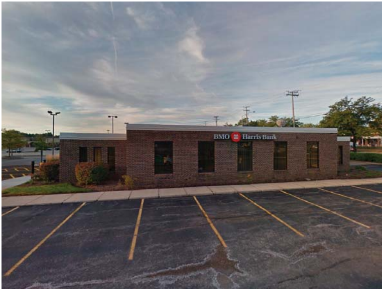
15 Site two Palantine Road to west.
