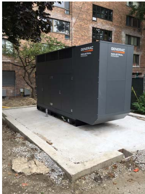
Existing Site Conditions
