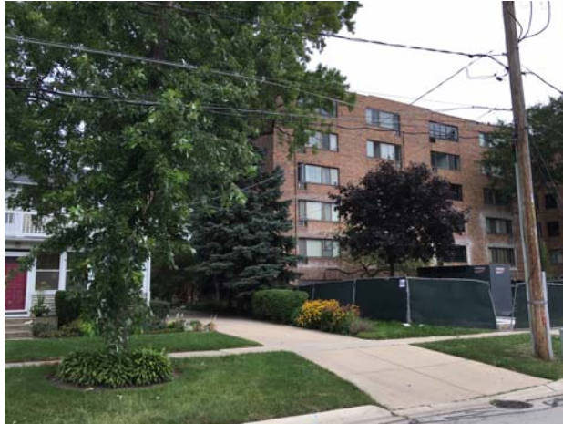
Existing Site Conditions
