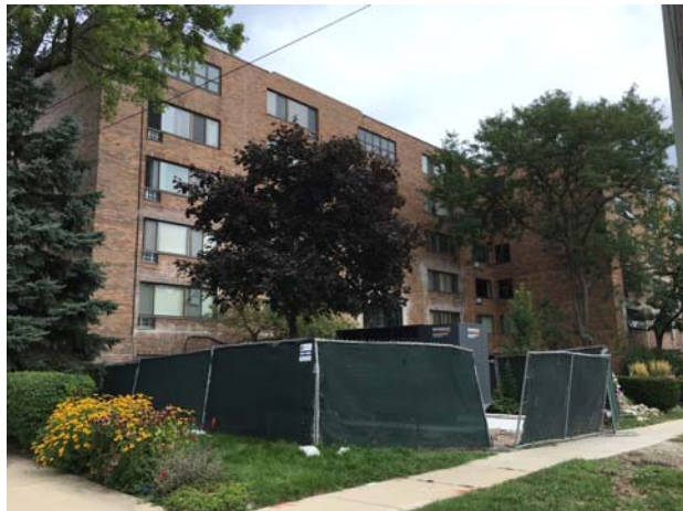
Existing Site Conditions
