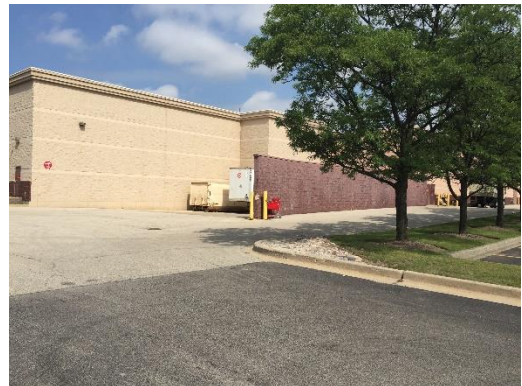
Figure 6: Existing truck dock and trash compactor screen wall
