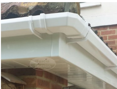
Gutters, Fascia, Columns:
