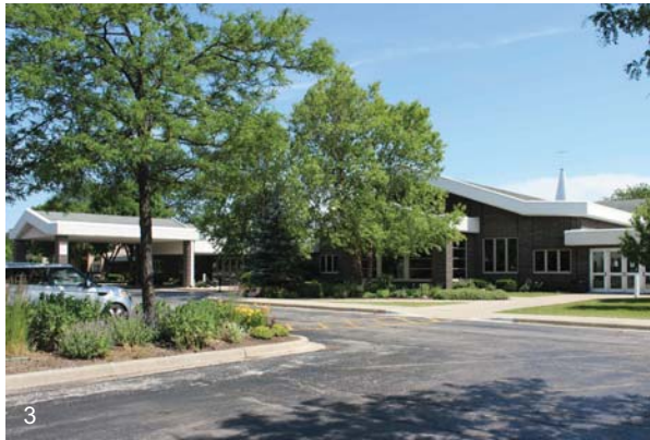
3 HURLEY CENTER - NORTHWEST ELEVATION
