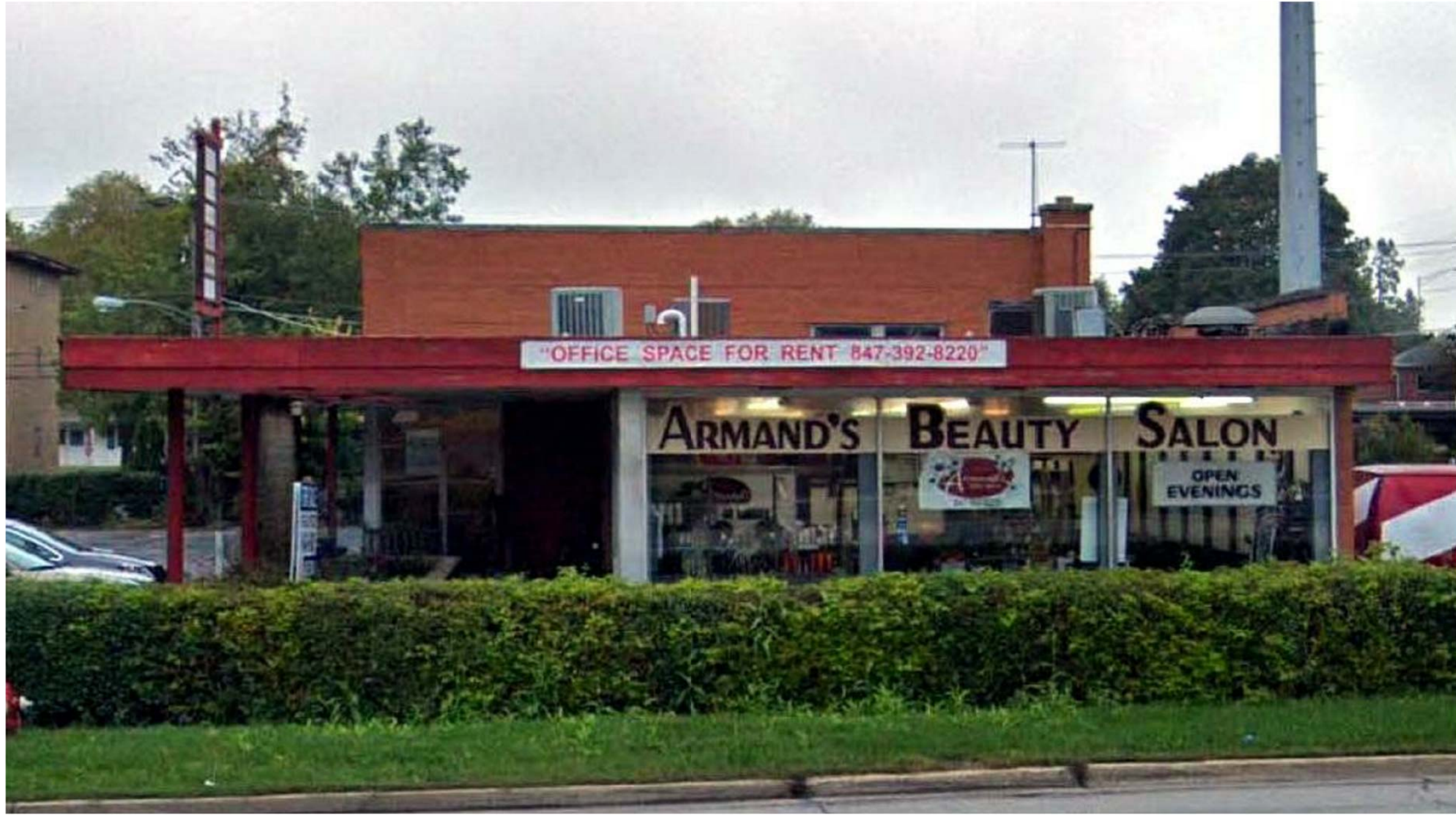
EXISTING EAST VIEW 12" = 1'-0"
