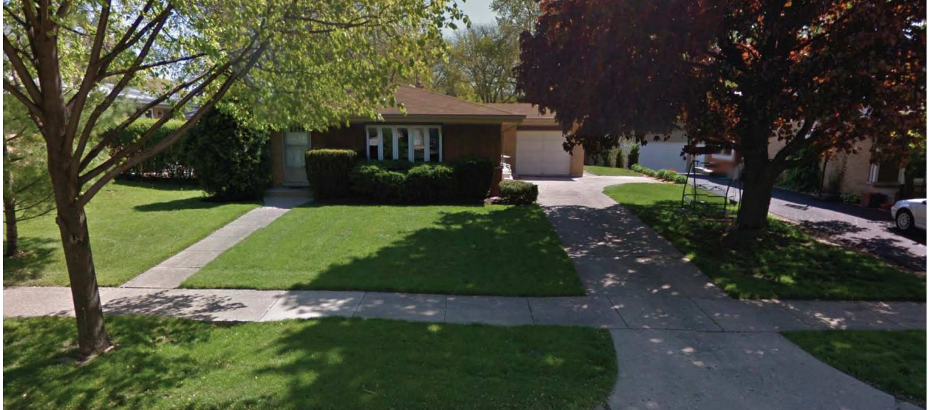
Photograph of Existing Structure
