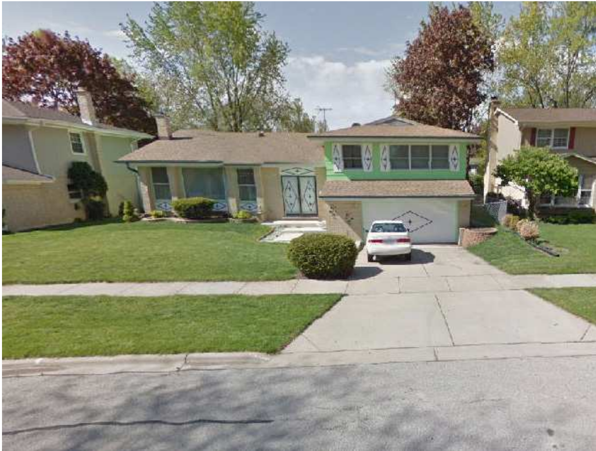
Photograph of Existing Structure
