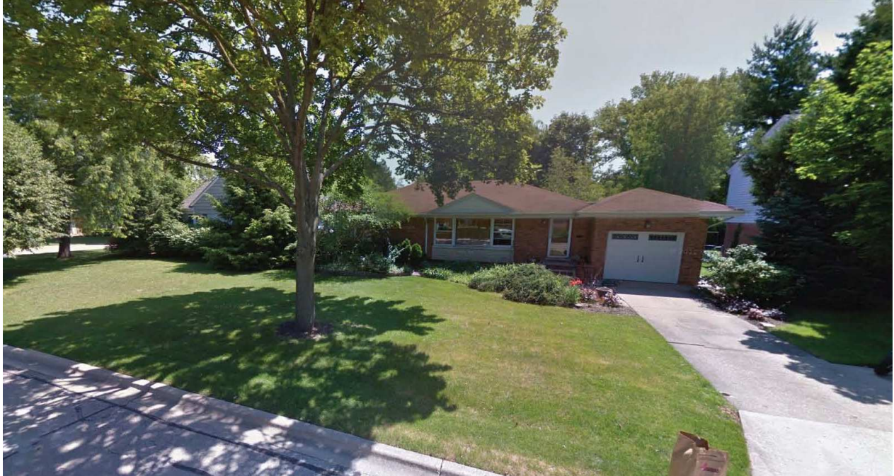
Photograph of Existing Structure
