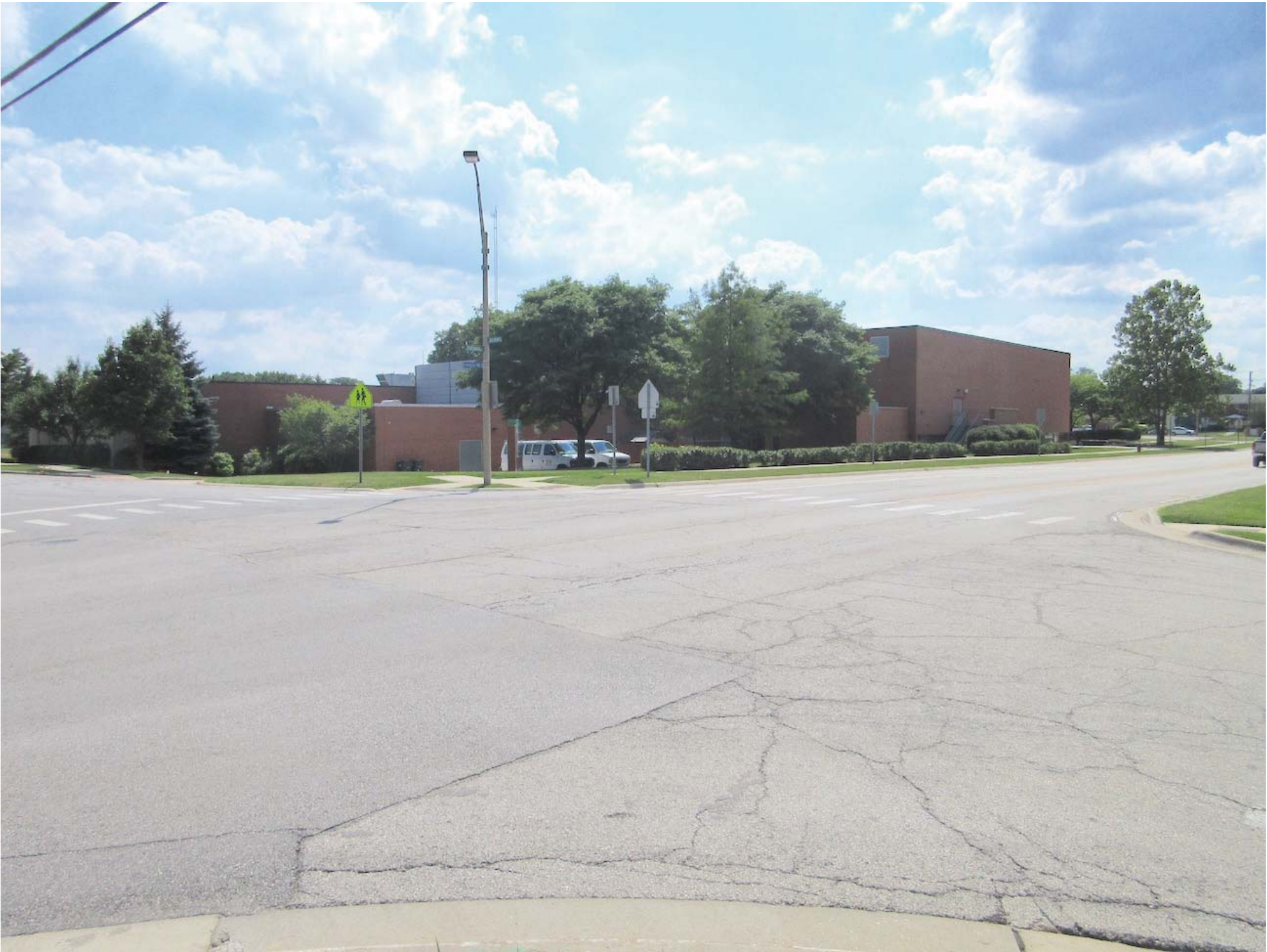
VIEW OF THOMAS MIDDLE SCHOOL FROM THE NORTHEAST
