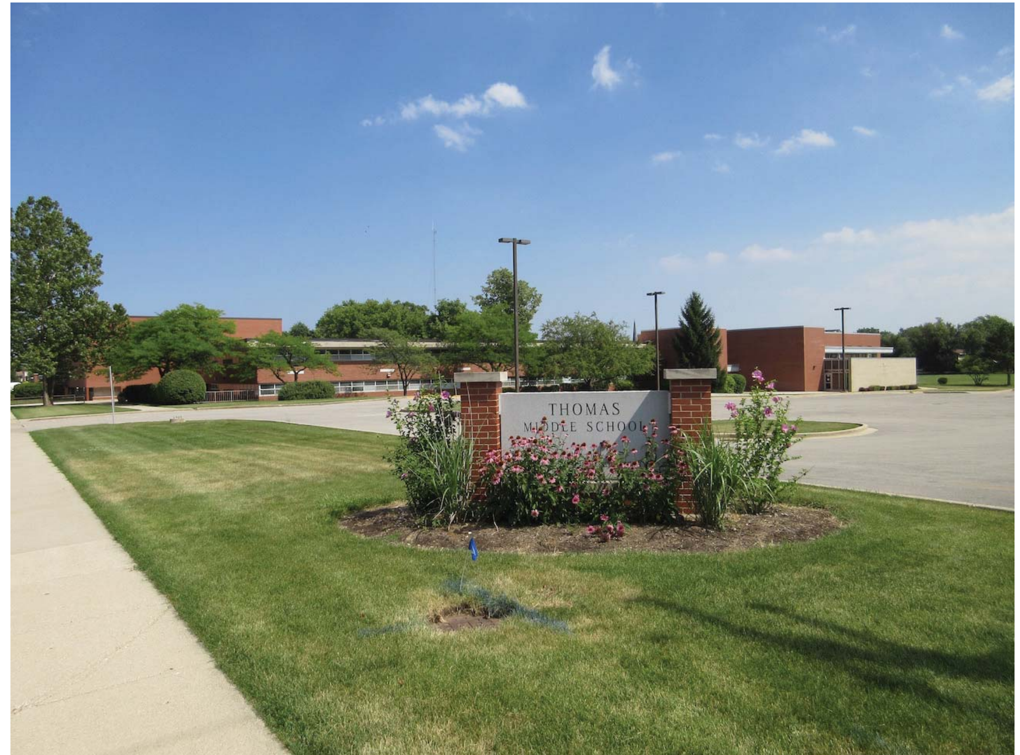
VIEW OF THOMAS MIDDLE SCHOOL FROM THE NORTHWEST
