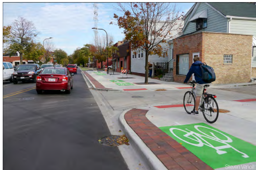
Figure 4.30 - Shared space for bicycles and pedestrians
