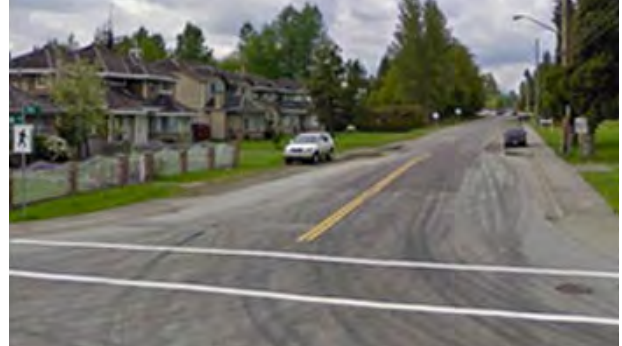
Figure 4.81 - Example A: Parallel Lines Crosswalk
