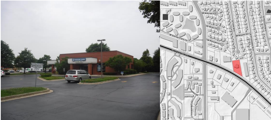
Parkway Bank – Right of the property (2)
