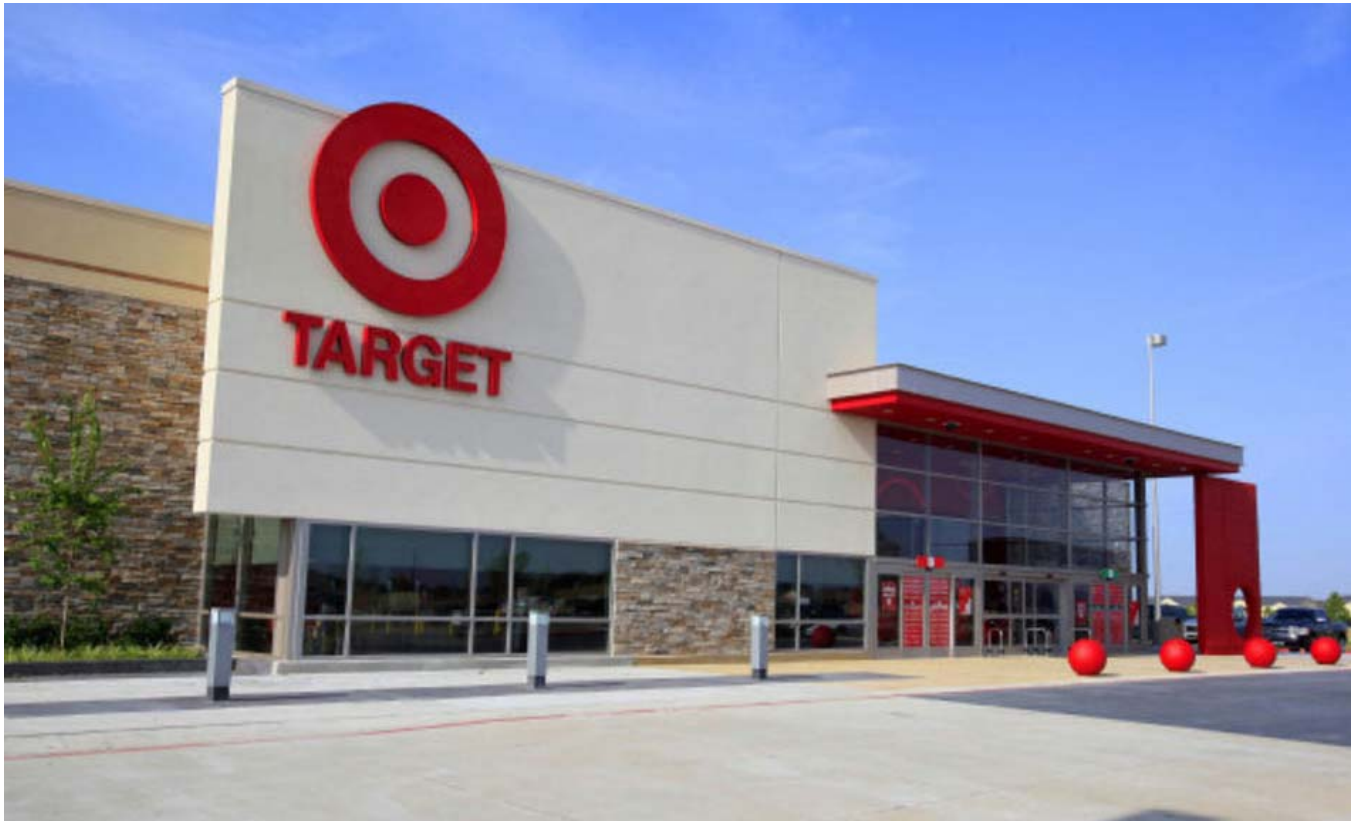
Photo 1. Example of a new Target store with bullseye logo projecting above the building wall.
