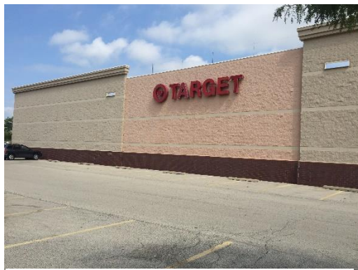
Figure 5: South side of Target
