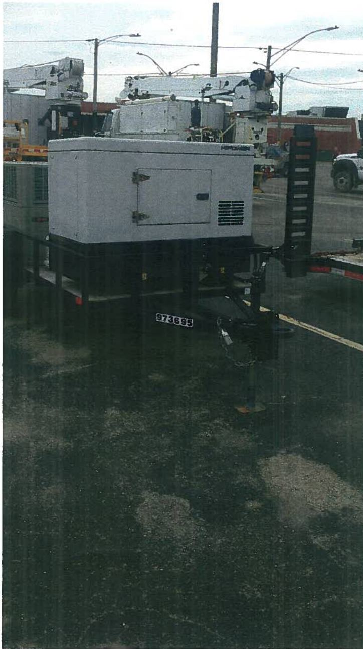
Air Conditioner Trailer
