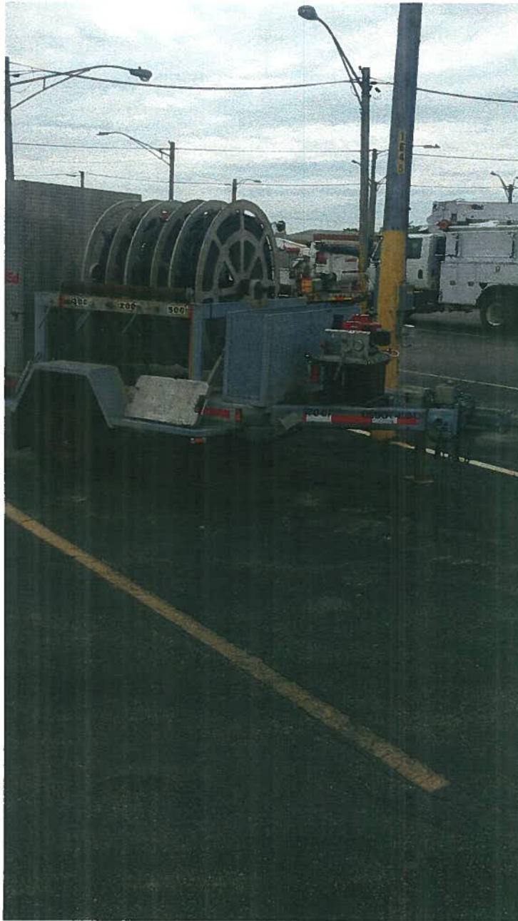
Temp Cable Cart
