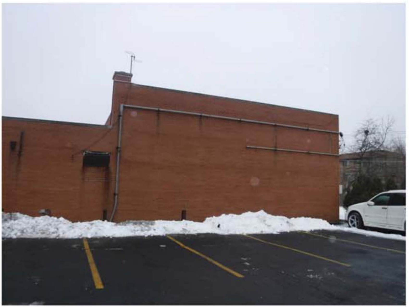
3 SOUTH WEST VIEW
