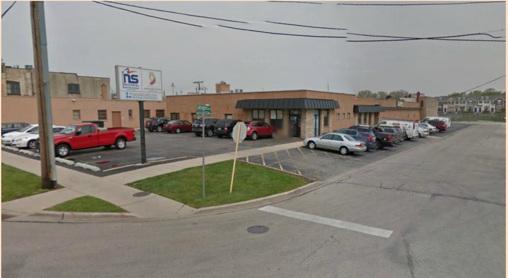
Looking Northwest from Kensington Road – Beverly Lanes Bowling Alley
