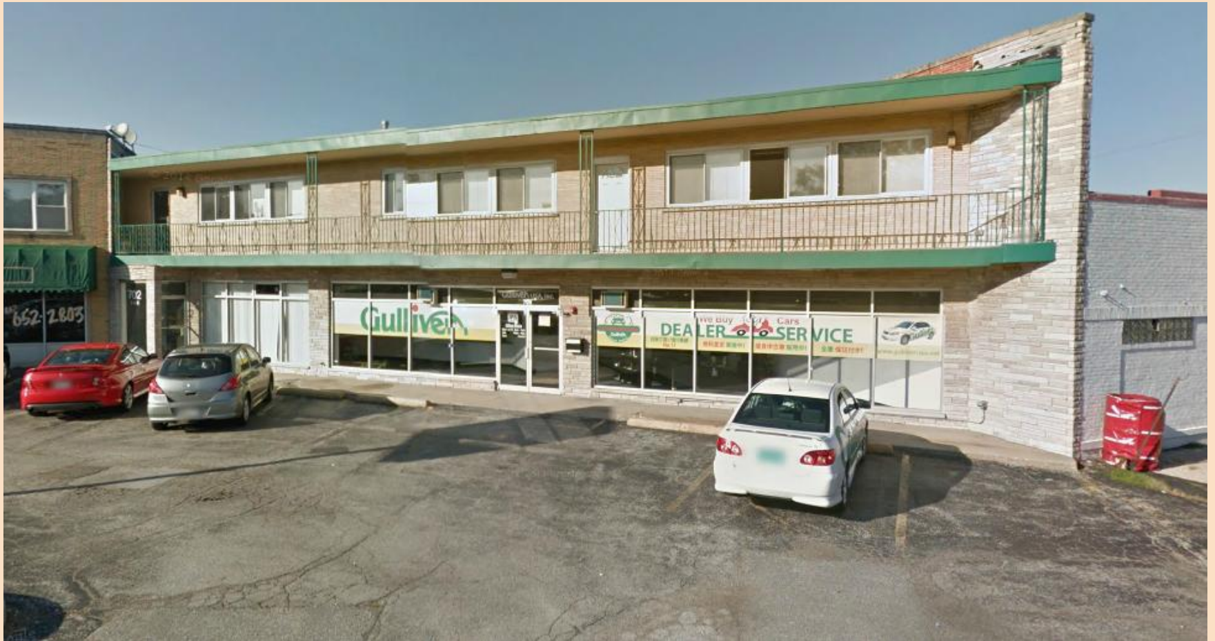
Looking North from Northwest Highway
