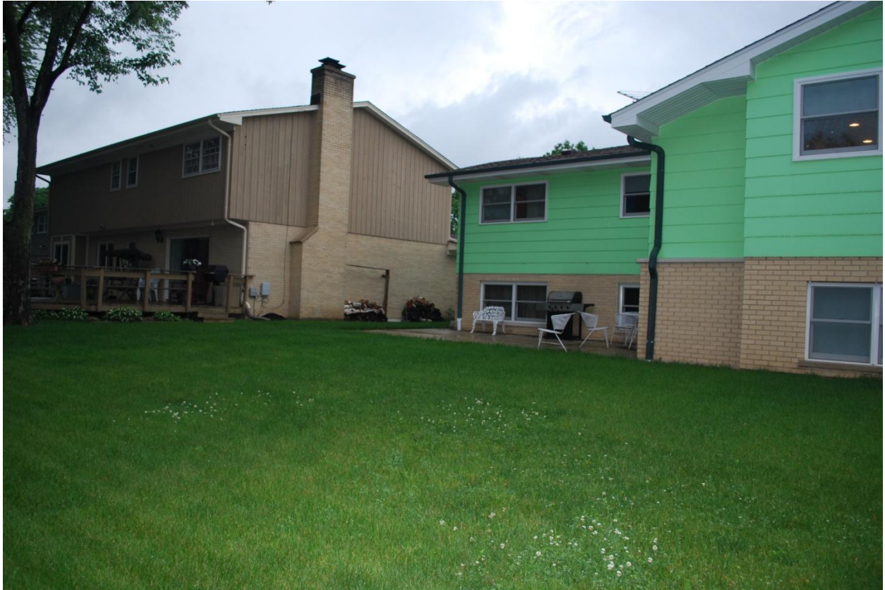
Rear of the existing house looking left
