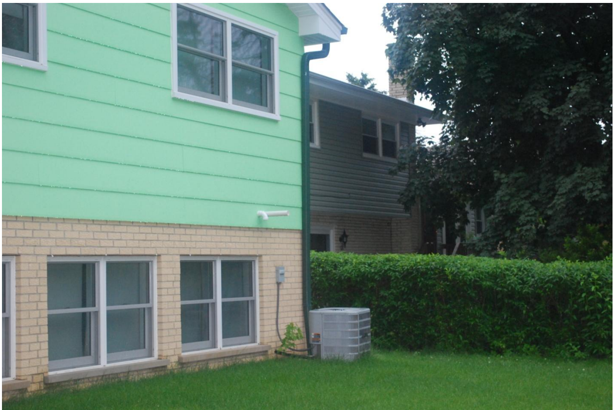
Rear of existing house looking to the right
