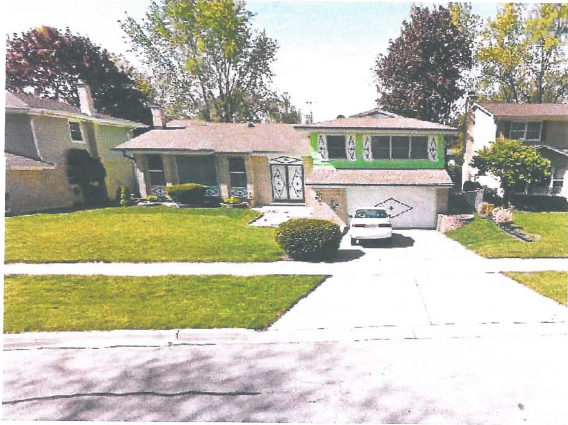
Photograph of Existing Structure
