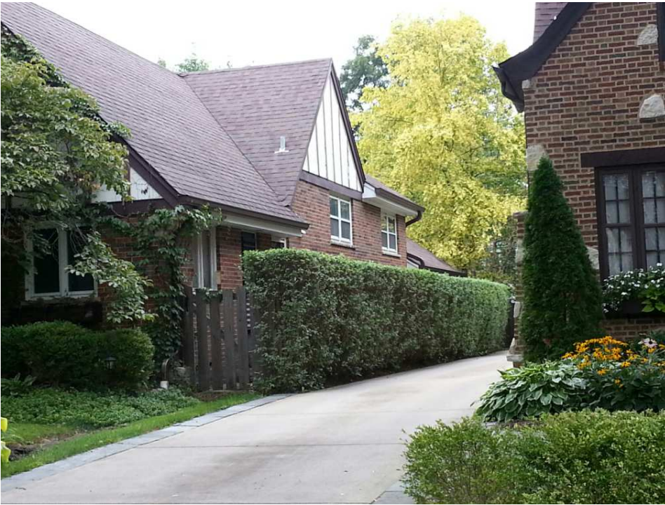
Photo 1. View of existing house from the street.
