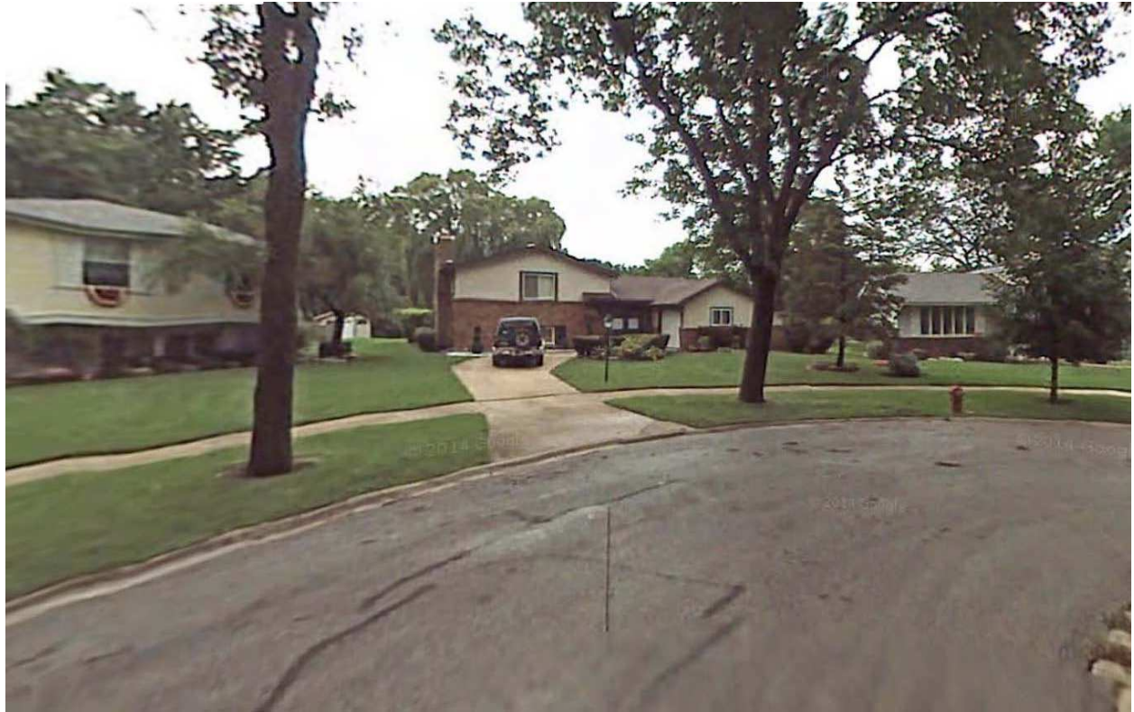
Photograph of Existing Structure
