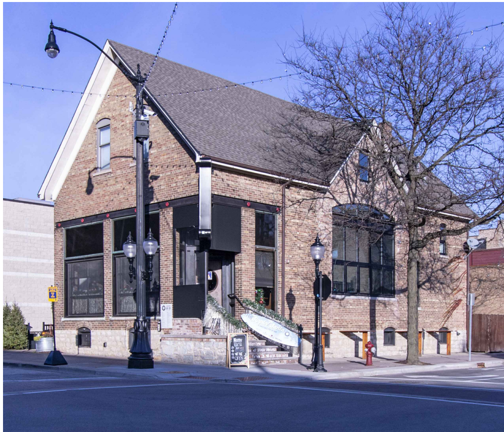
EXISTING FRONT OF BUILDING
