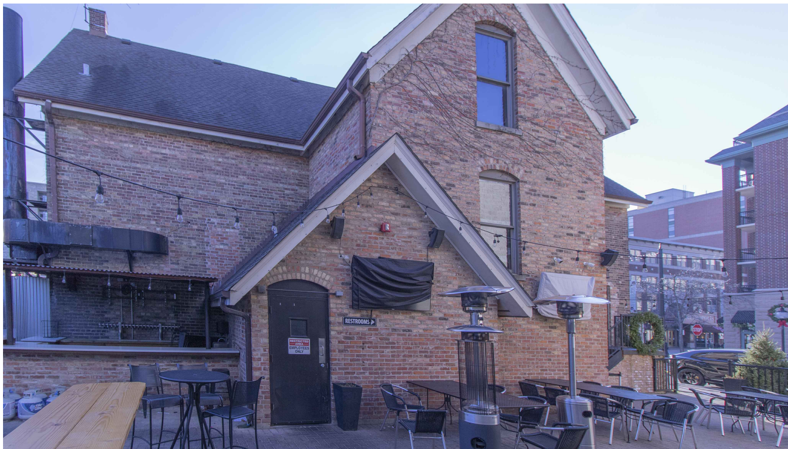
EXISTING REAR OF BUILDING - CANOPY LOCATION
