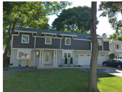
641 SOUTH BURTON PLACE (ACROSS-R)
