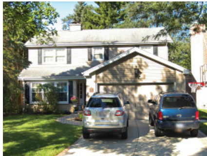
640 SOUTH BURTON PLACE (LEFT-2)
