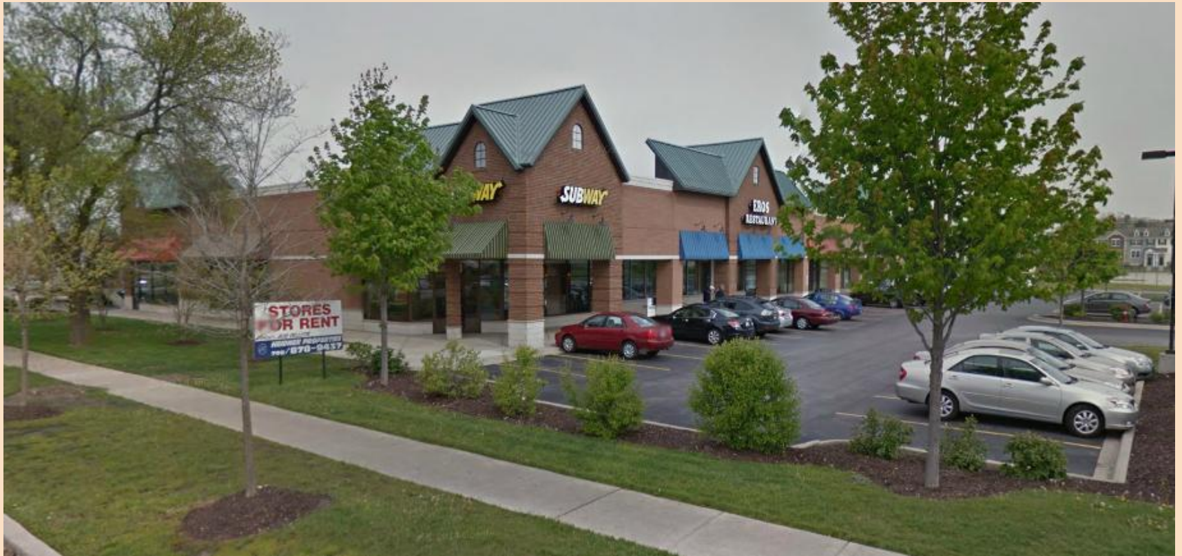
Looking Northwest from Kensington Road
