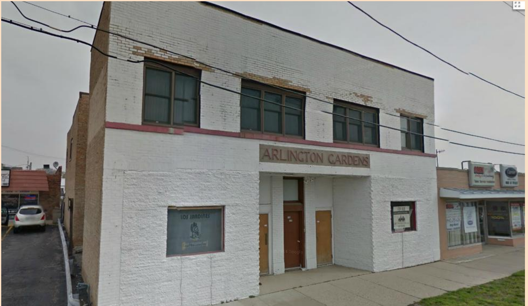
Looking North from Kensington Road
