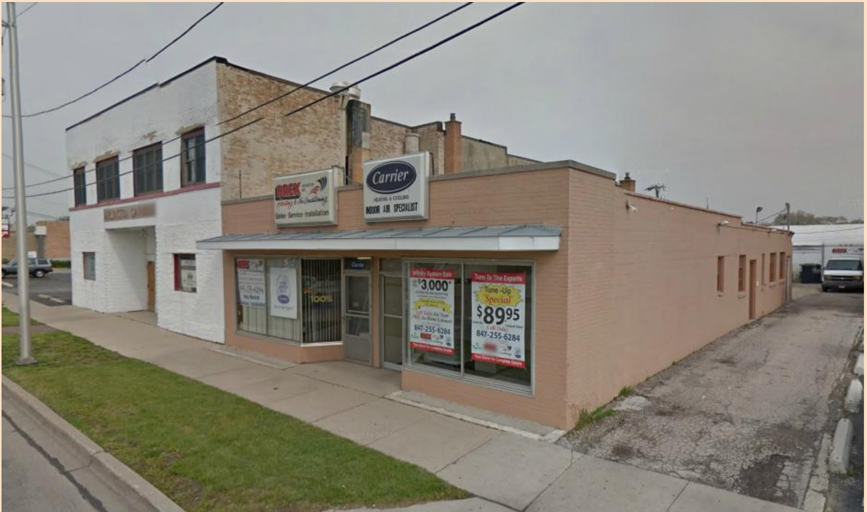
Looking Northwest from Kensington Road
