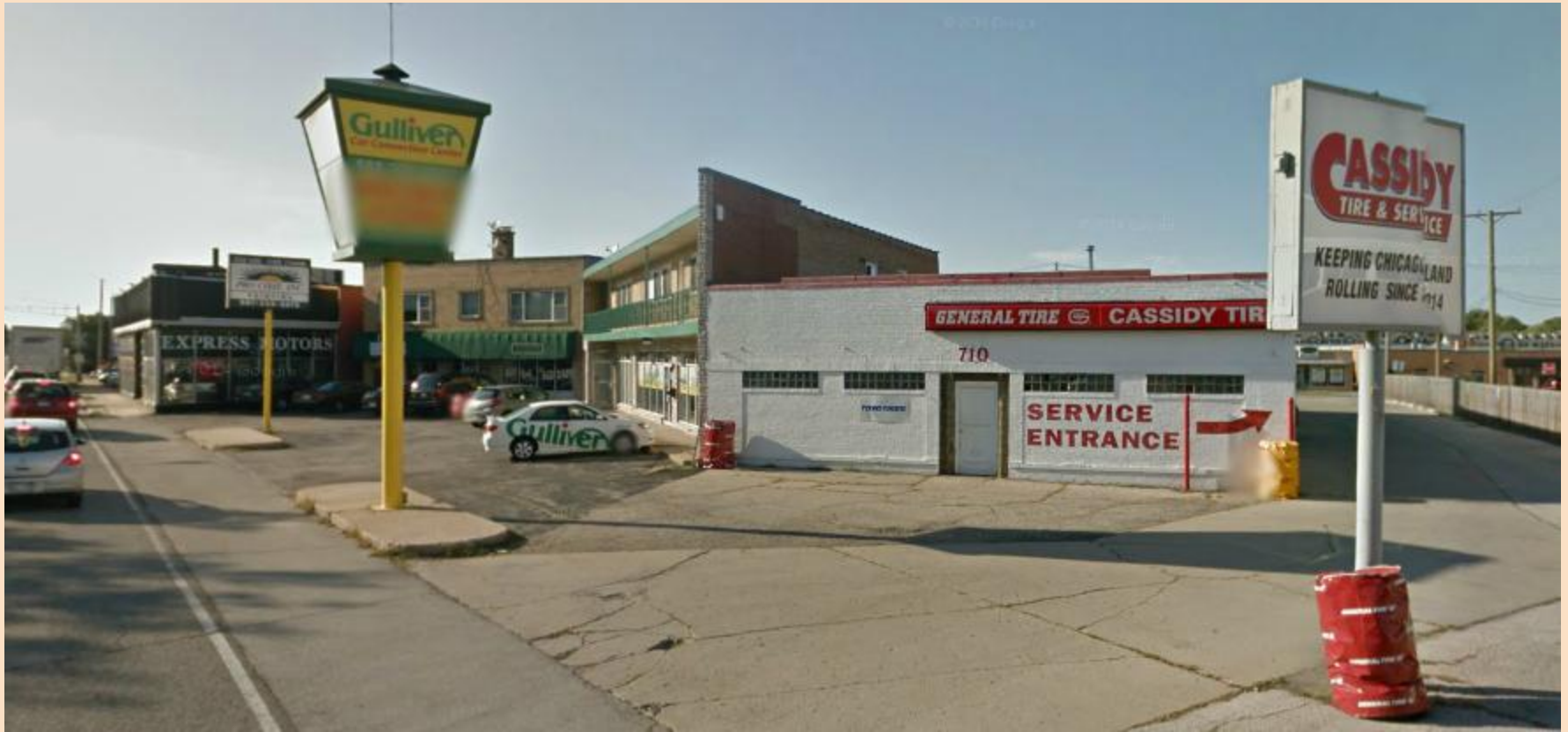
Looking Northwest on Northwest Highway – Cassidy Tire & Service
