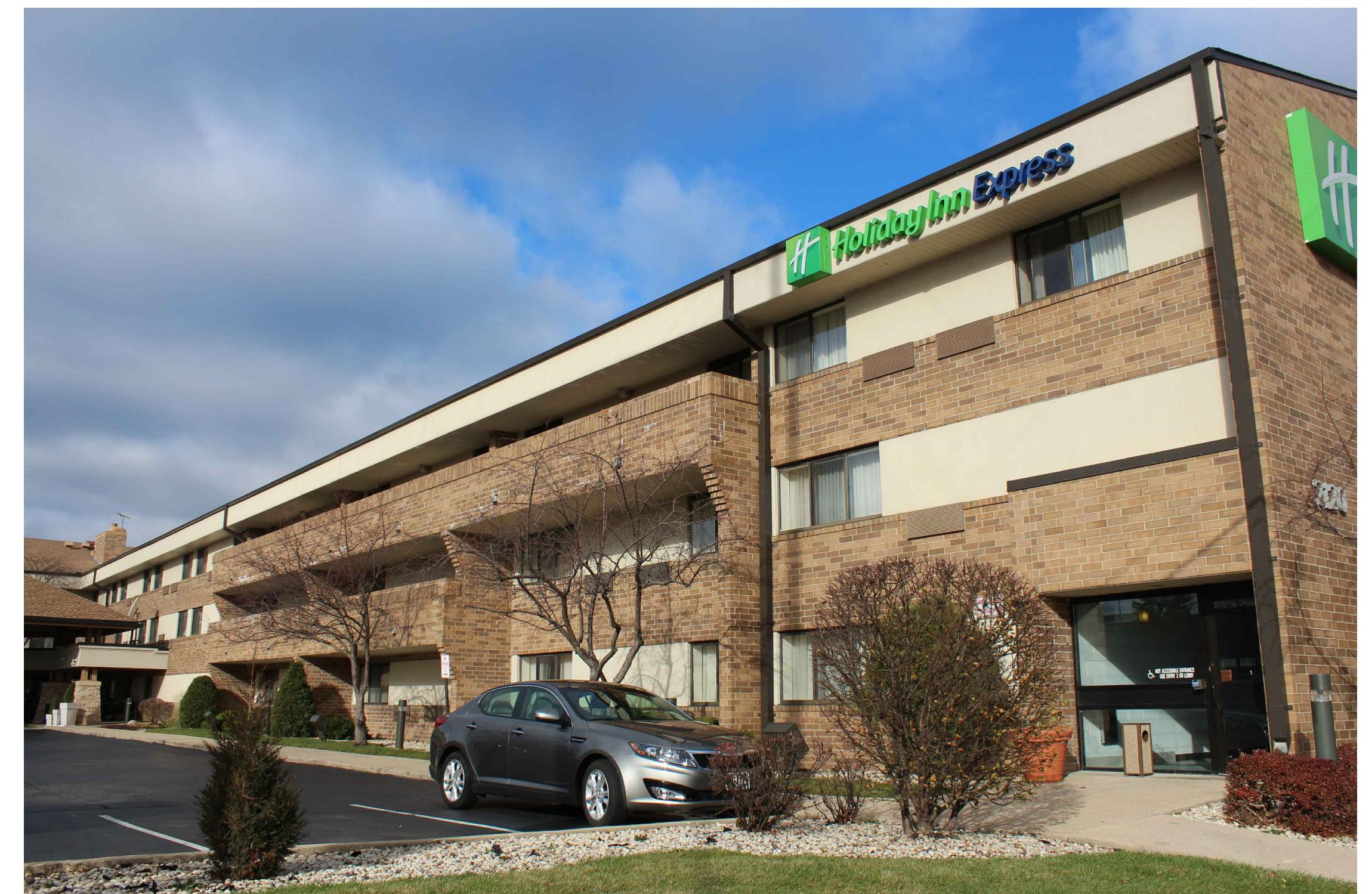
4 EXISTING SOUTHWEST VIEW SCALE: N.T.S.
