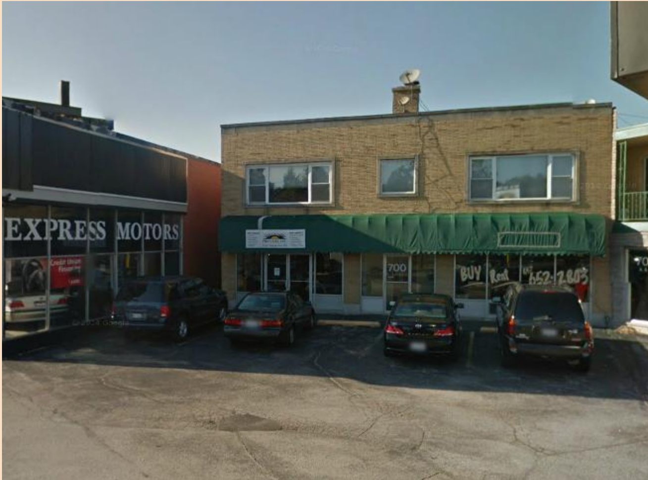
Looking North from Northwest Highway
