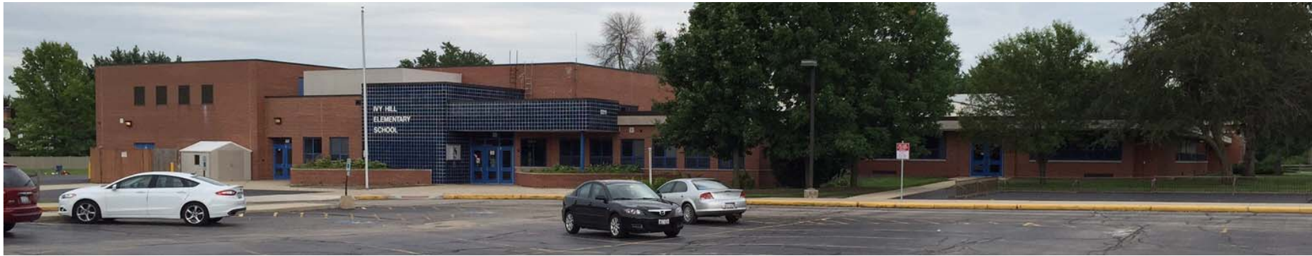
VIEW OF SCHOOL - FACING NORTH
