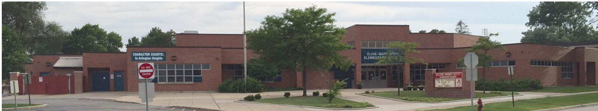
VIEW OF SCHOOL - NORTHEAST CORNER
