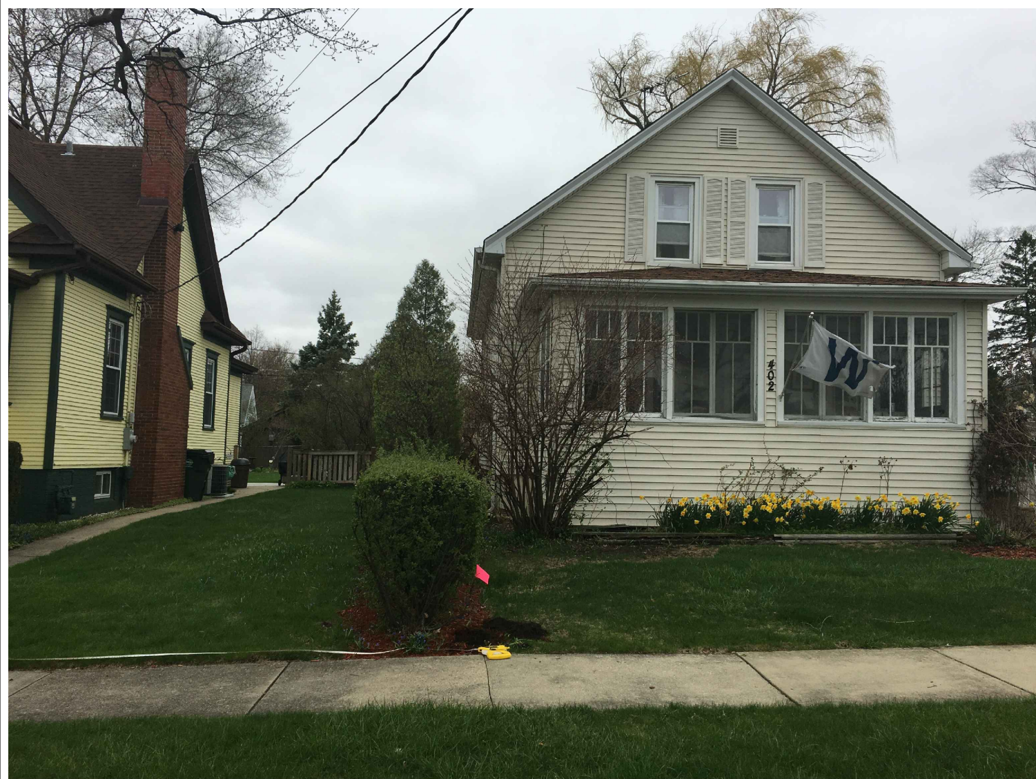
EXISTING SINGLE FAMILY RESIDENCE AND DETACHED GARAGE
