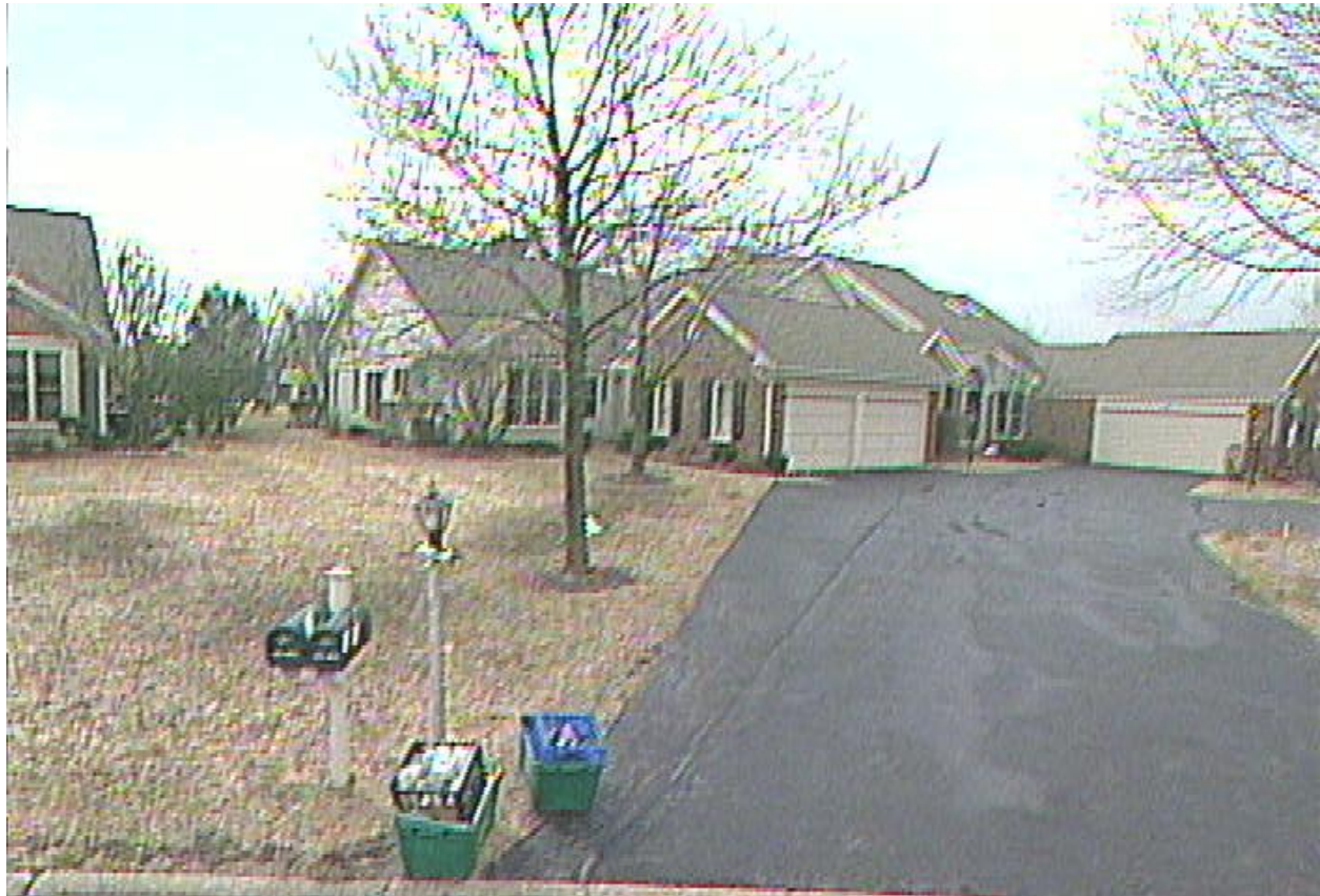
Photograph of Existing Structure
