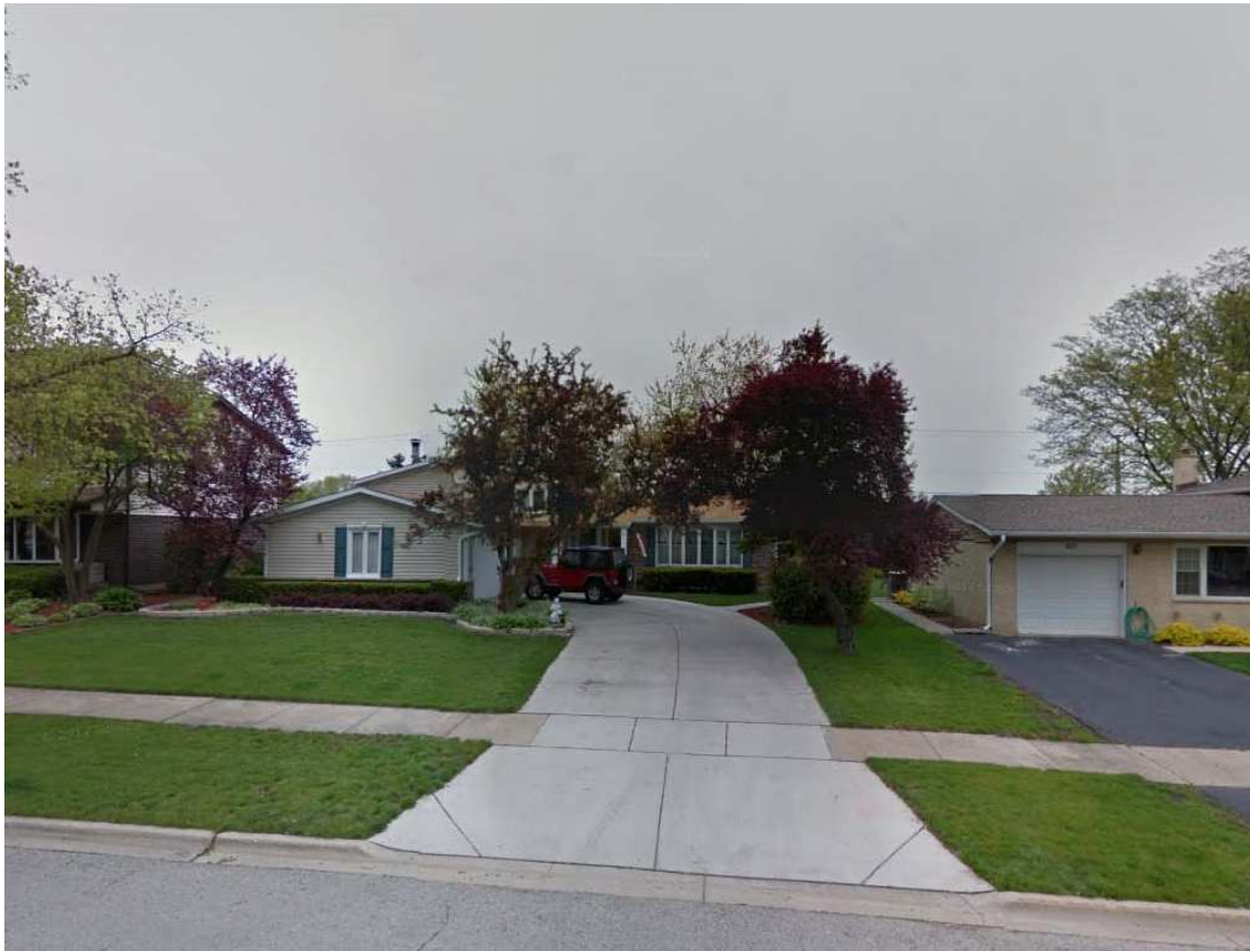
Photograph of Existing Structure
