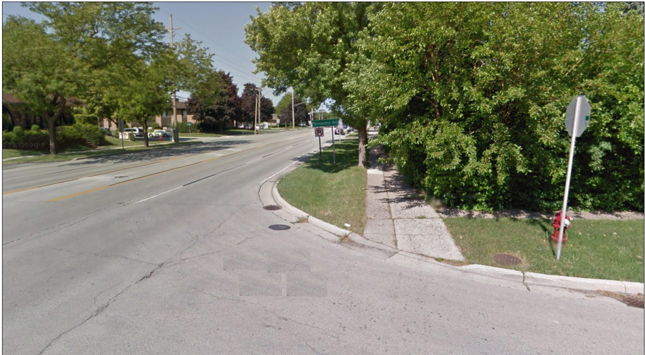
Figure G1 - Current conditions of sidepath (retrofitted from sidewalk) along Central, at Walnut. Although along the framework route, it is not appropriate as a bikeway, due to pavement condition and encroachment of vegetation.
