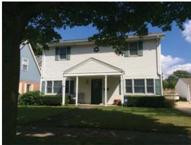
Property to Left 2 913 N Hickory Ave
