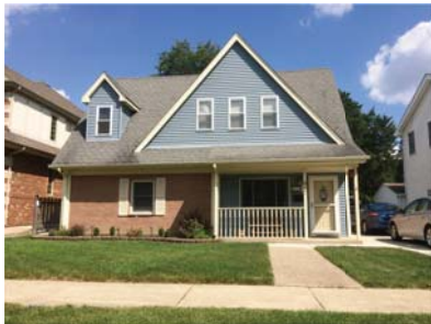
Property to Left 3 917 N Hickory Ave
