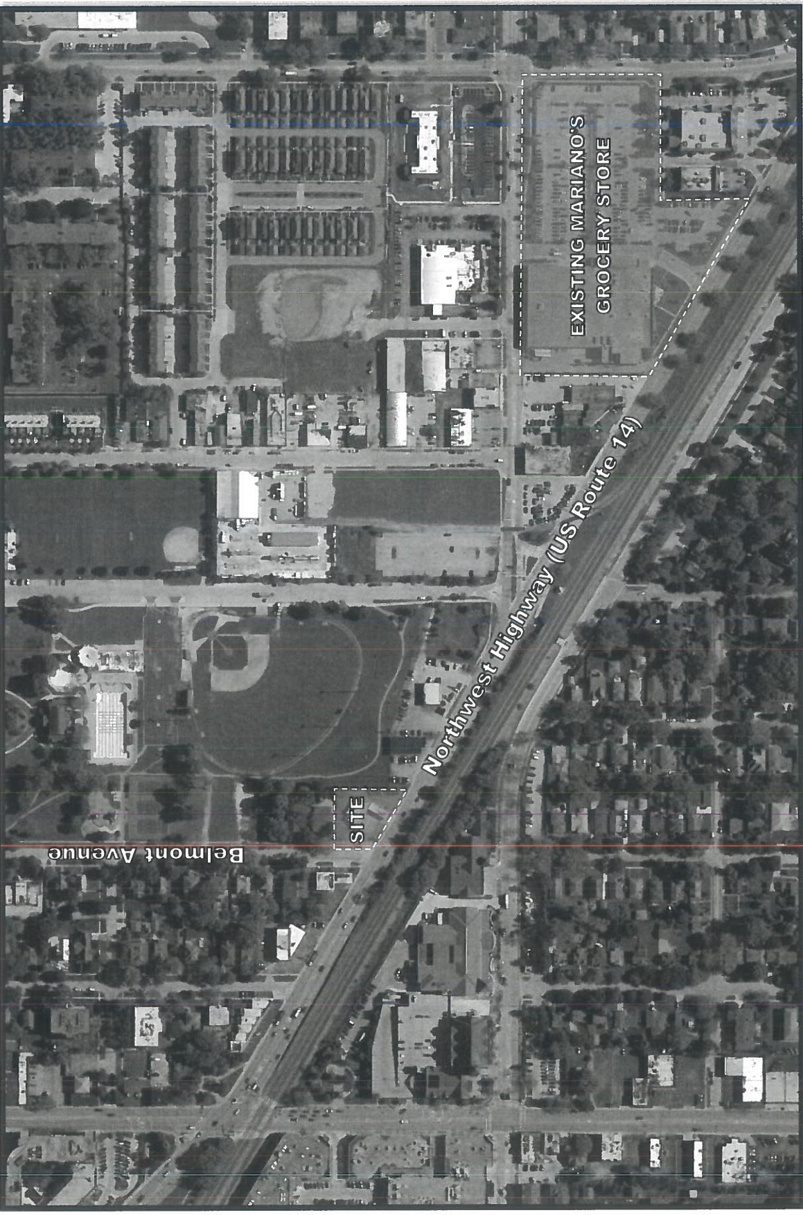
Aerial View of Site
