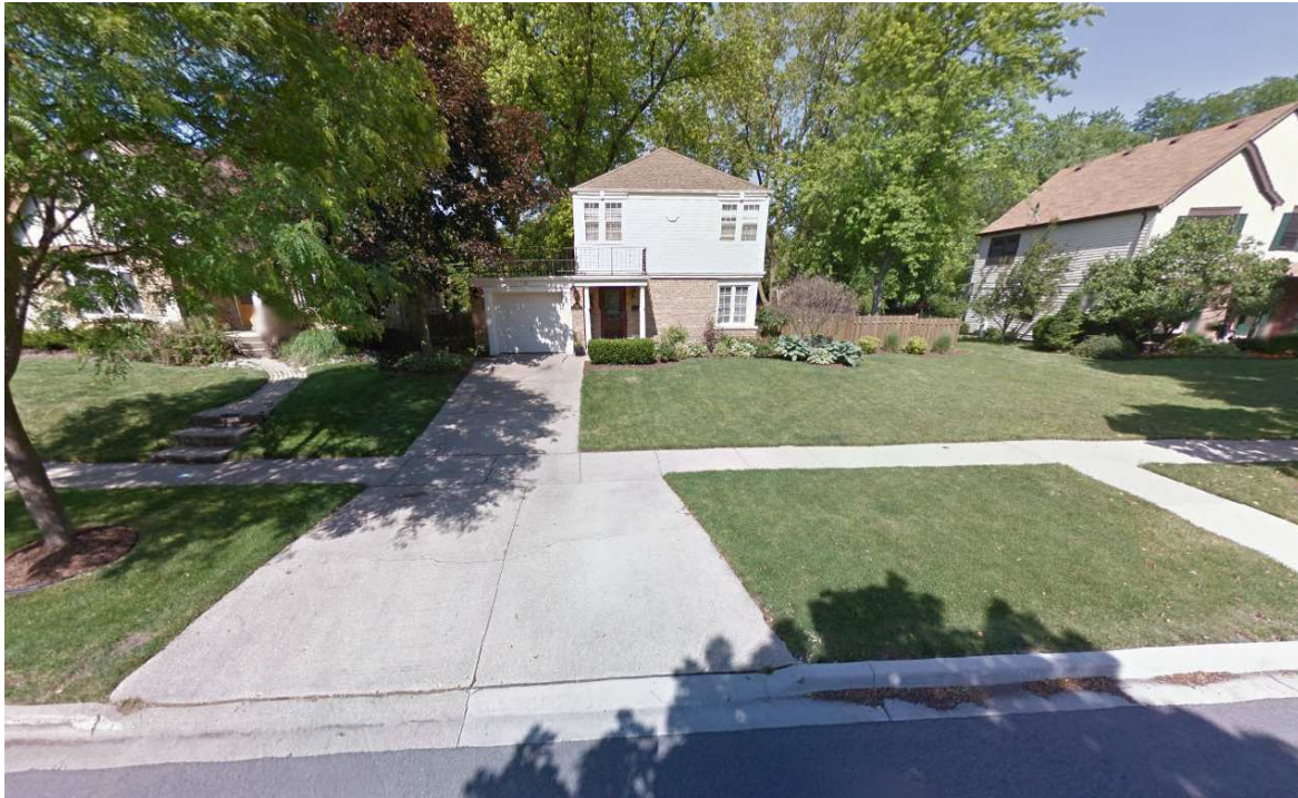
Photograph of Existing Structure
