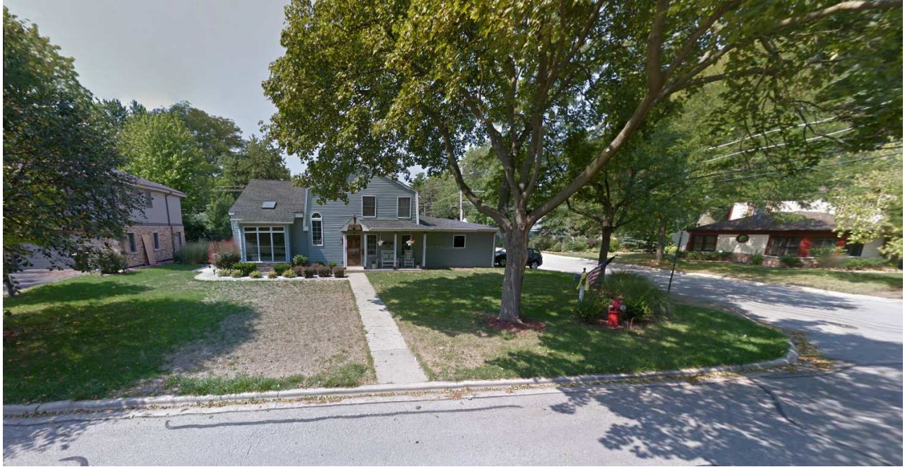
Photograph of Existing Structure
